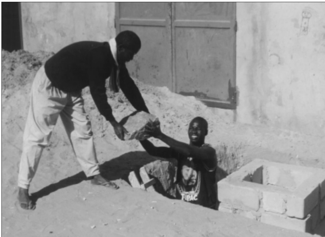
Construction of septic tanks in Yeumbeul, Senegal © G. Domenach-Chich
