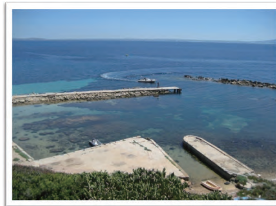
Current situation of the port Zembra
