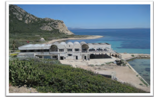
Shelter in Zembra installed in the 60
