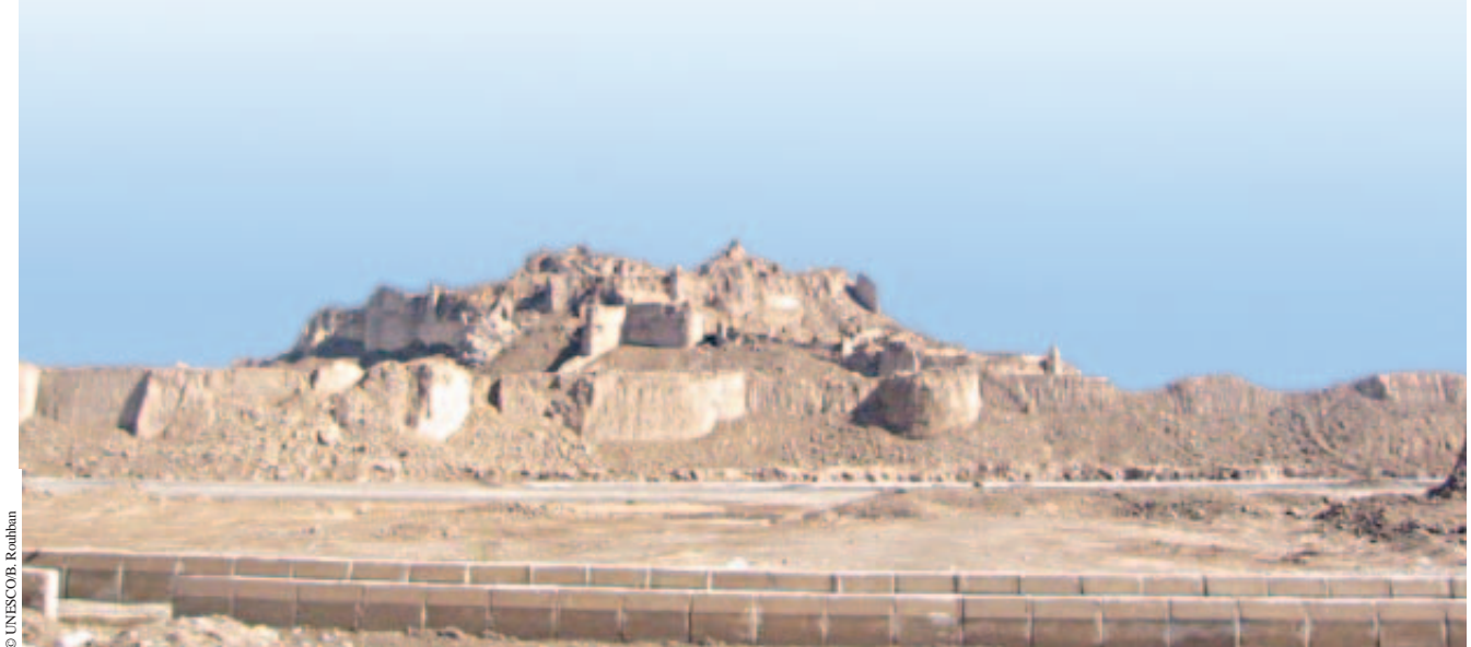
The badly damaged Bam Citadel (Arg-e-Bam)
