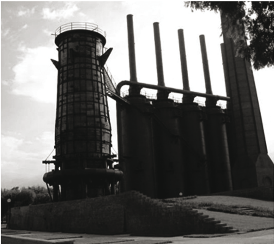
Blast furnace no. 1 and the set of hot-blast stoves
