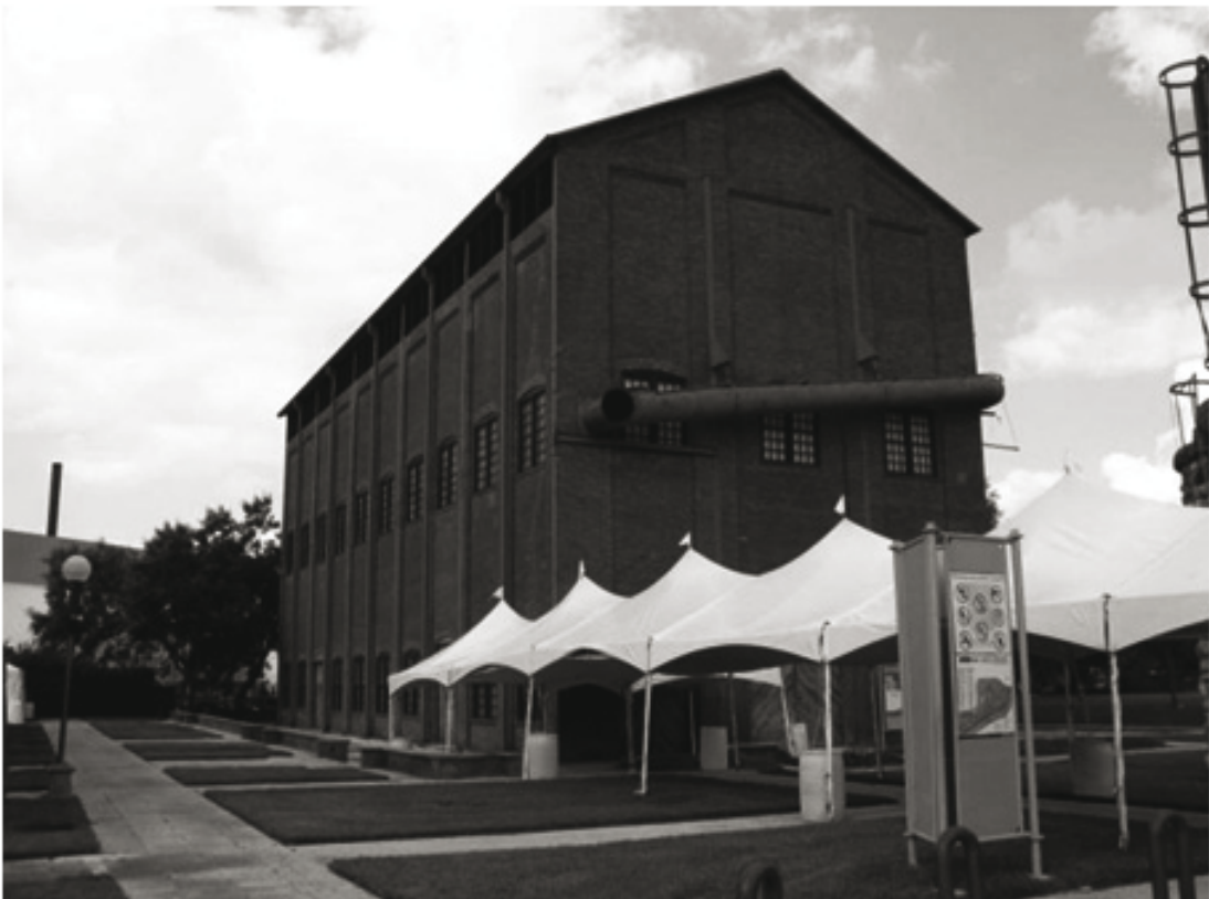
The compressor building after restoration
