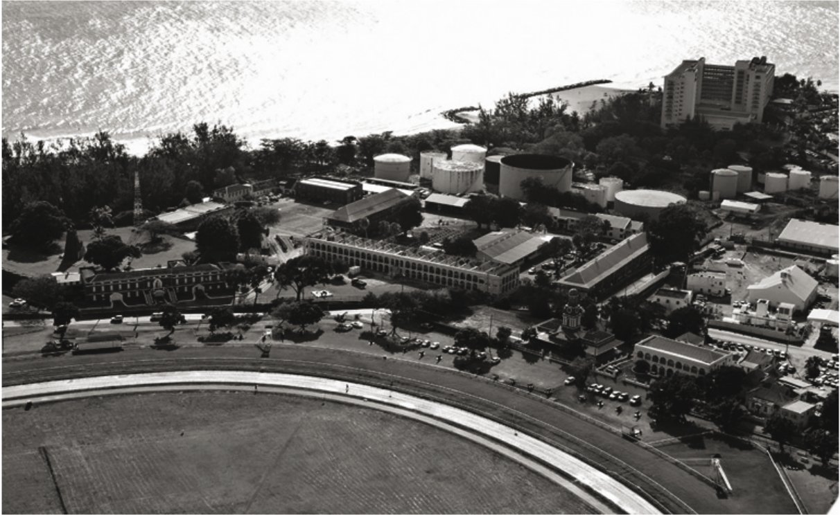
Drill Hall, Stone Barracks and Main Guard, the Garrison
