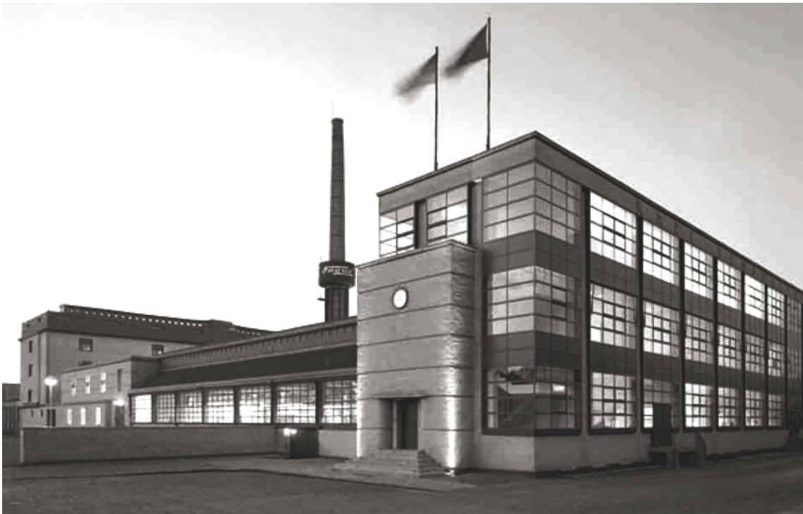
South-western view of the main building
