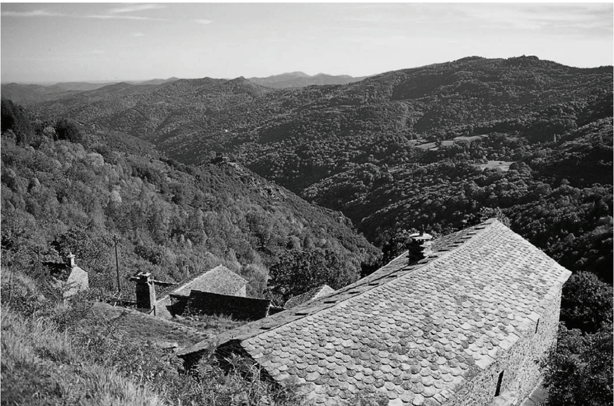
Roof in shell-shaped slates
