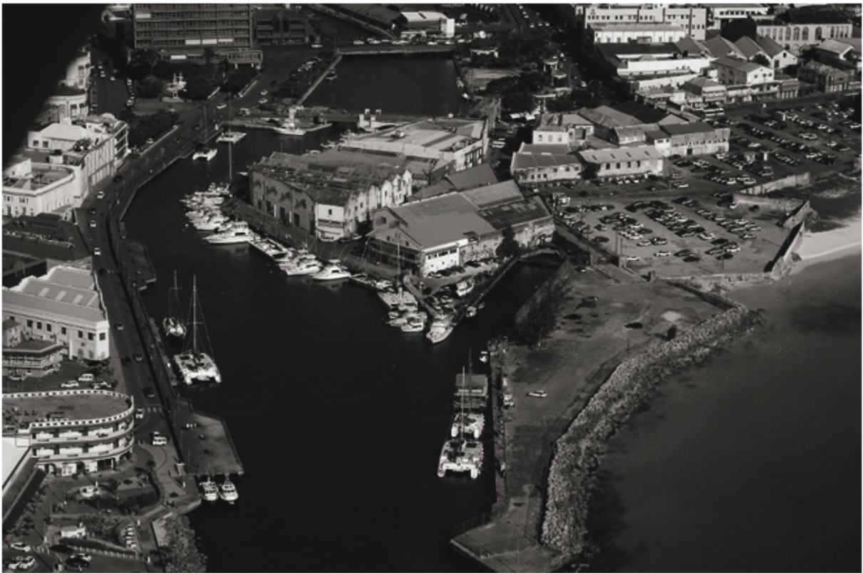
Warehouses and Screw Dock at Pier Head
