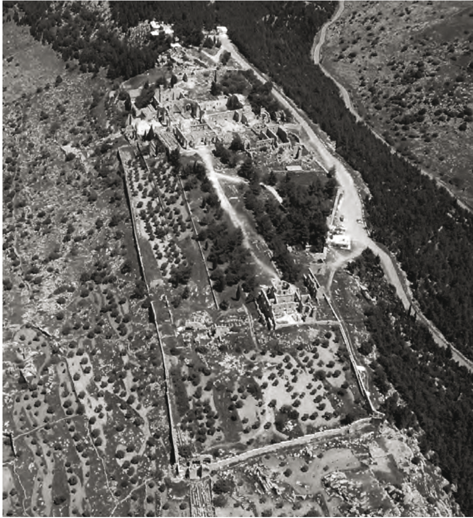
Aerial view of Saint-Simeon site
