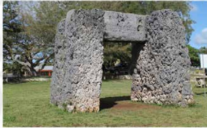
Fig. 5: Ha'amonga 'a Maui Trilithon – the crossing stone is most vulnerable to earthquake
