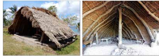
Cyclone Shelter Nakamal in Nuna Island © K. Masuda
