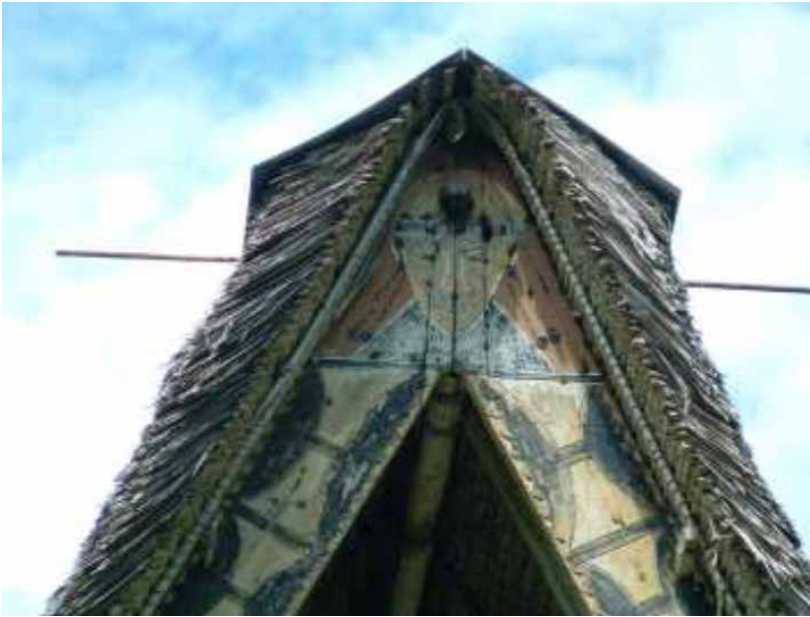
Fig 2: Roof thatching Airai Bai
