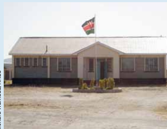
The school administration block
