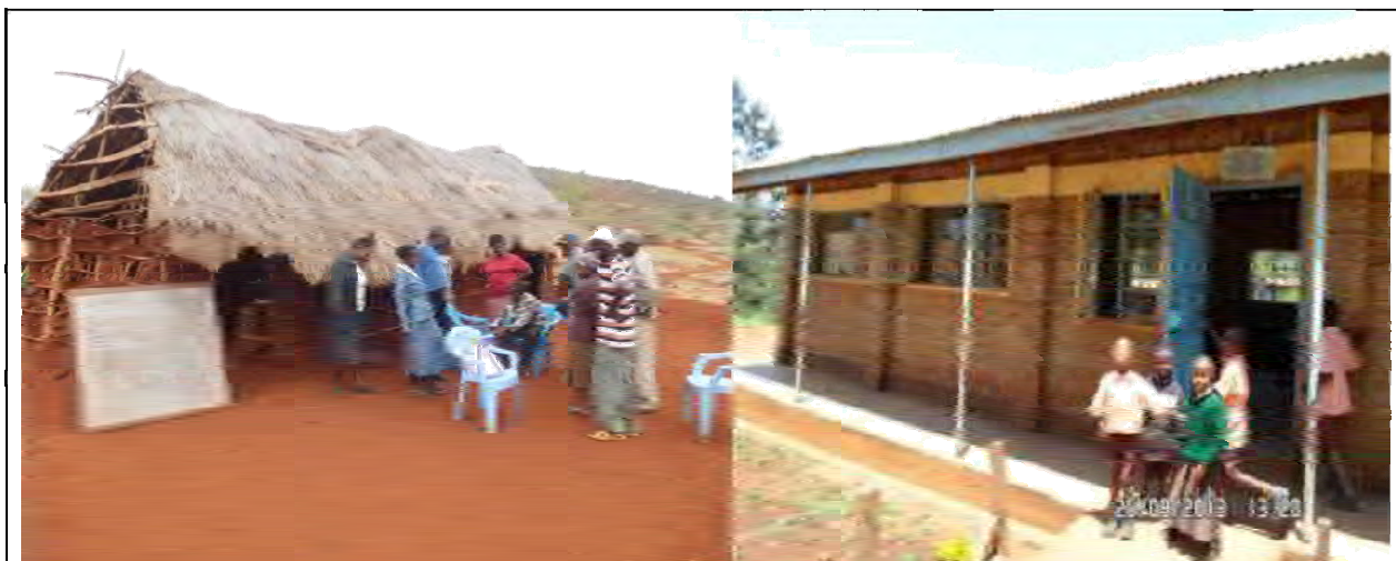
Note: The photos above show ECCE facilities before the renovations were carried out and after.
