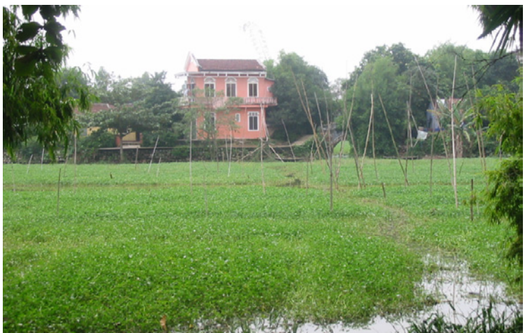
Non-traditional building amidst the historic hydrologic heritage of the Hué Citadel
