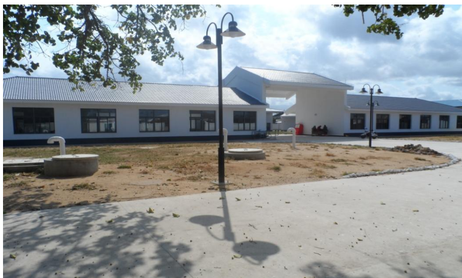
New primary school constructed at Mwanakwerekwe West District.
