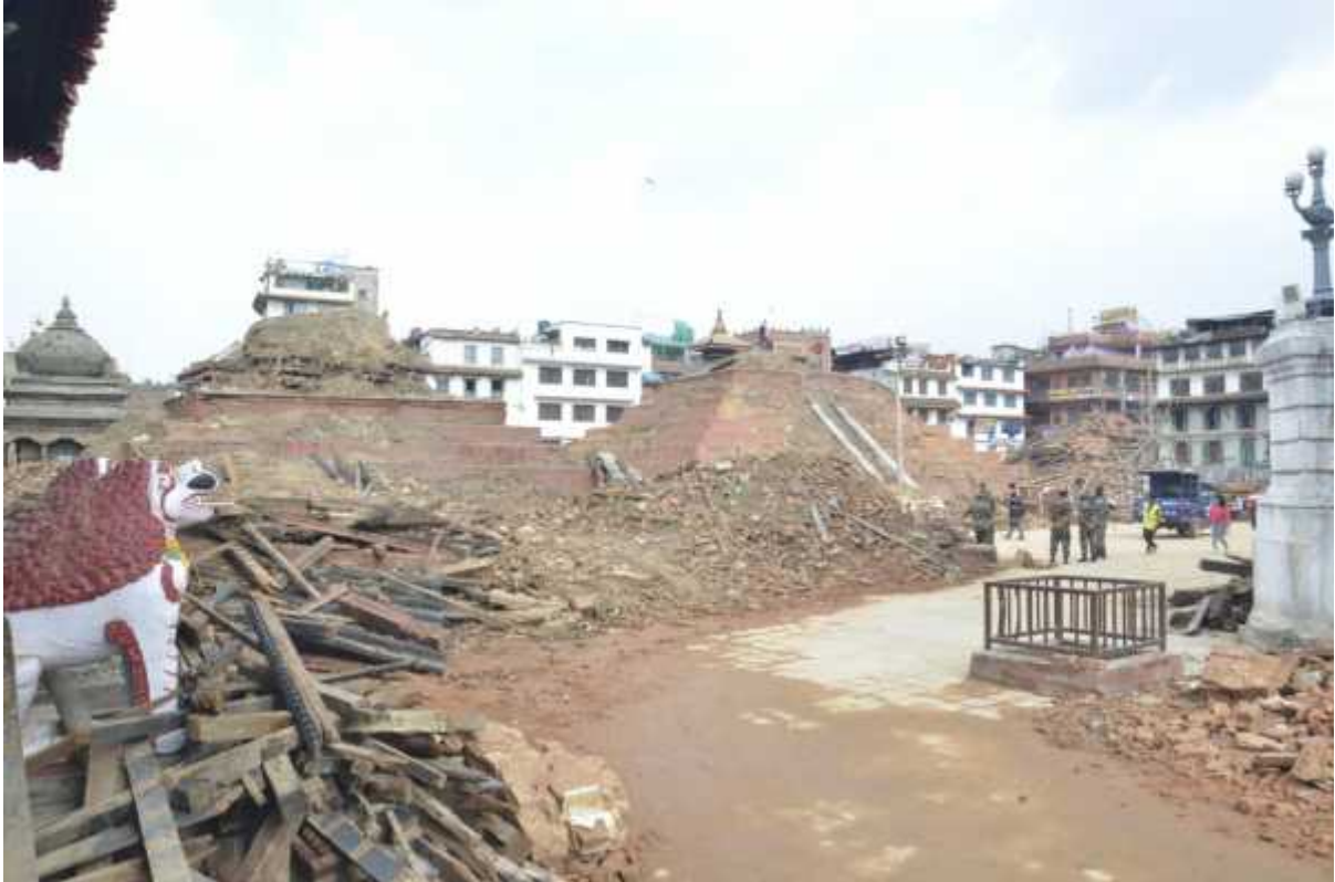
Pun Dega, Maju Dega and Narayan Temple (After Earthquake)
