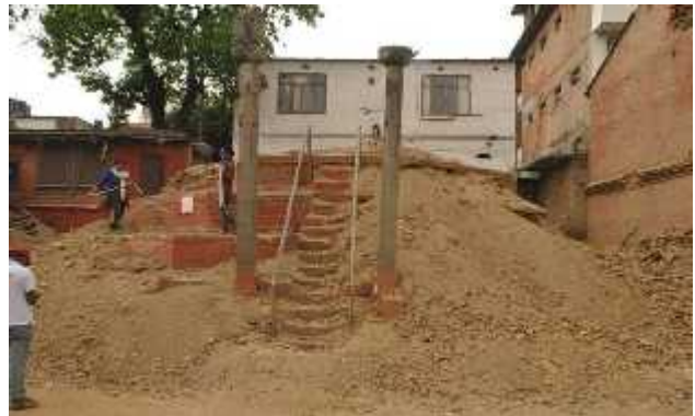
Chyasilin Dega (After earthquake)
