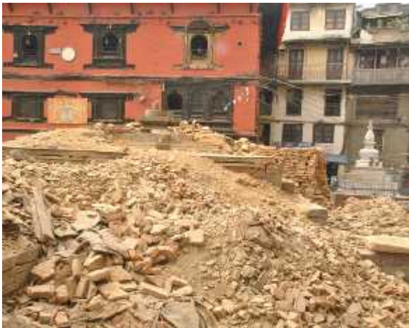
Nau Dega (After earthquake)
