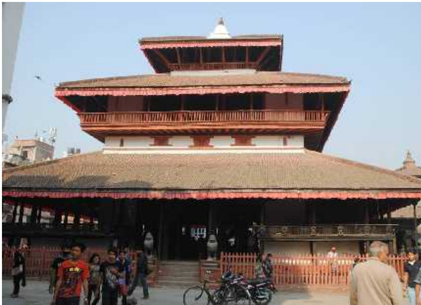
Kasthamandapa (Before earthquake)
