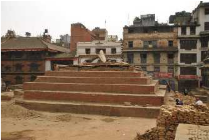
Pun Dega (After earthquake)
