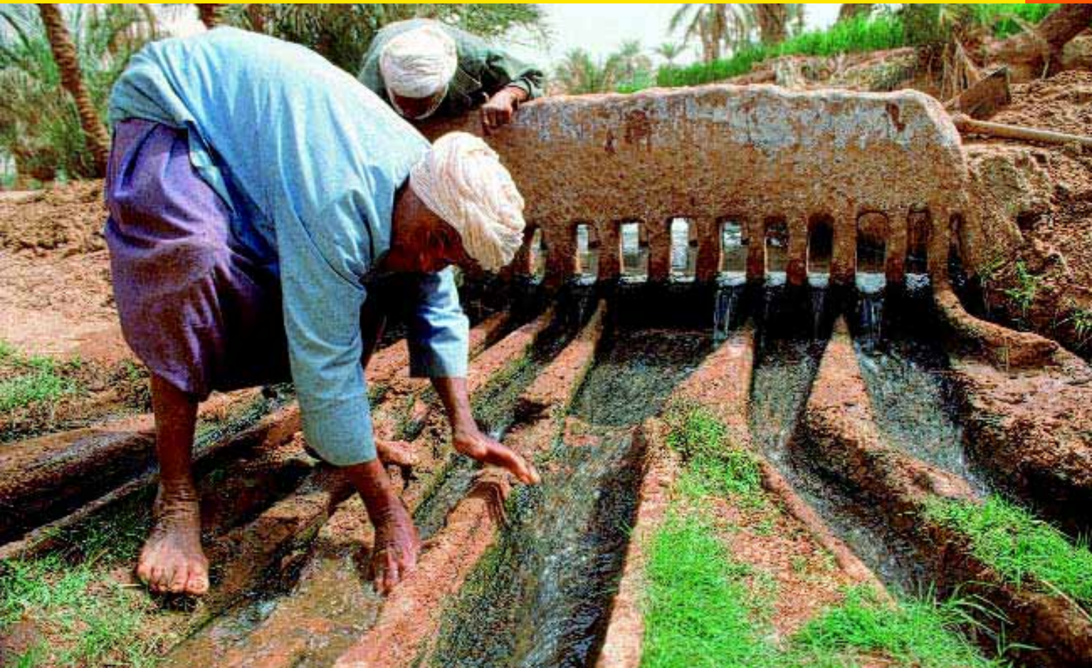
Photo 2. The kesria permits water distribution in the oasis.
