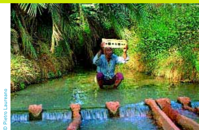
Photo 1. The foggaras system distributes water throughout the oasis.
