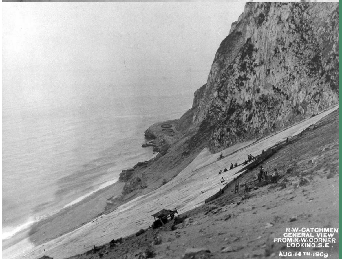
FIGURE 2.98 Almost the entire (14 ha) dune was covered by corrugated metal sheets that were laid between 1903 and 1961 for the purpose of collecting rain water. Image (above) shows extension to waterworks, July 1925 and (below) works in 1909. Gibraltar Museum.
