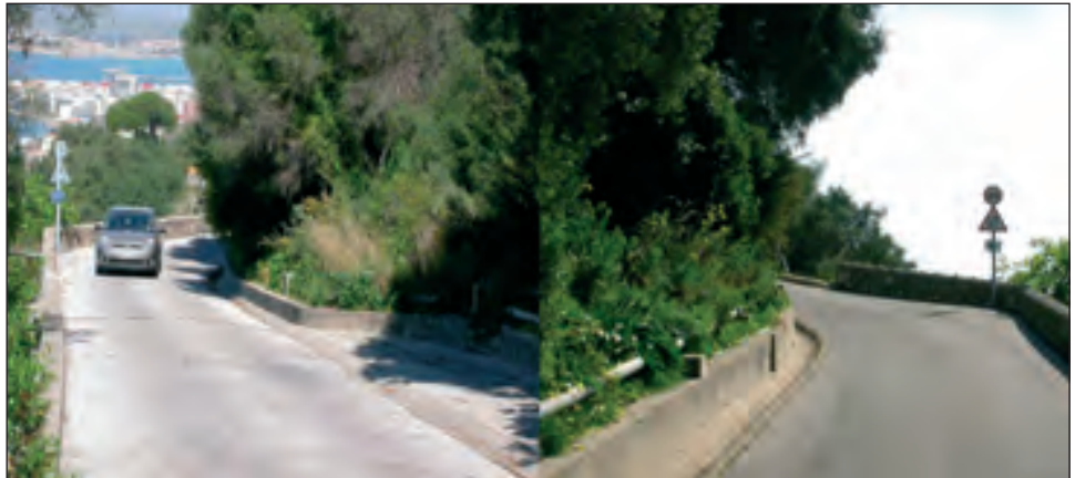
Figure 2. Engineer Road bend, looking north.
