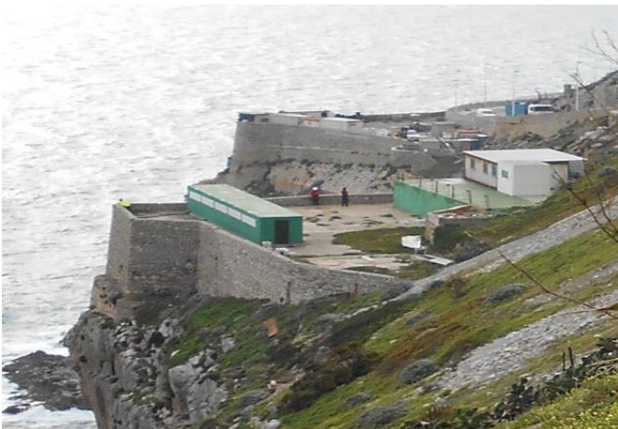
↑Photograph 6: 3 rd Europa Advance Battery from the north before refurbishment, in 2014, with 1 st and 2 nd Batteries to the top.
