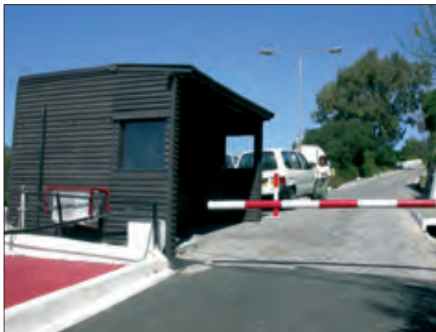
Figure 1. Second ticket booth at Jews' Gate, with bollards protecting the structure.
