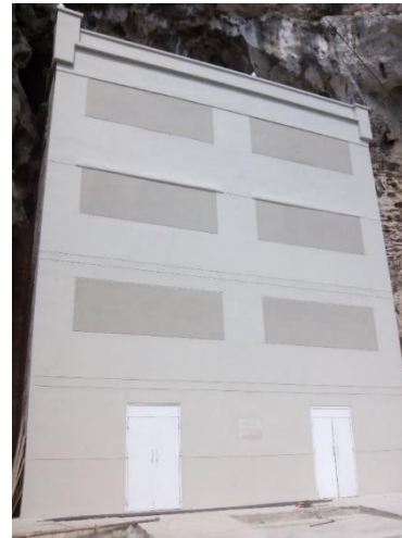
↑ after renovation of the façade
