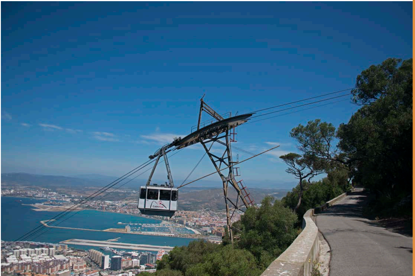
FIGURE 5.8 Visits to the Mediterranean Steps are on foot, either completely or via the cable car to the Top of the Rock.
