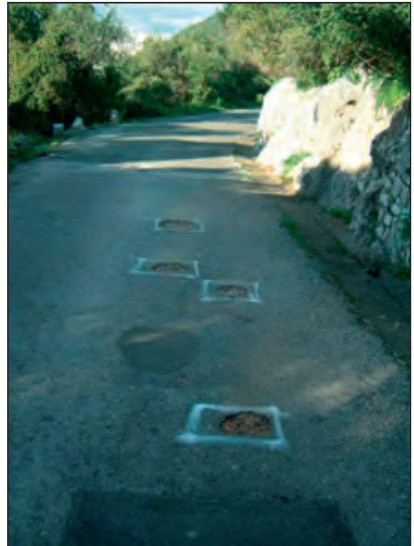
Figure 4. Potholes along Queen's Road remained marked by a white or yellow, square perimeter for a long time before being filled.
