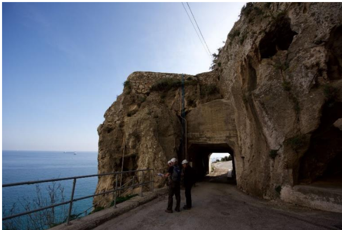
4 th Europa Advance Battery from the north. The battery wall is visible on top of the Second World War tunnel cut through to Monkey's Cave Hospital and AROW Street. The access steps to the sea caves descend from just below the battery behind the railings.
