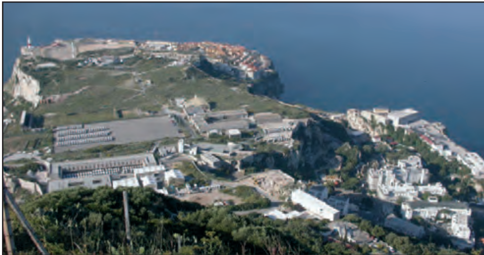
Figure 11: View of part of the South District of Gibraltar.
