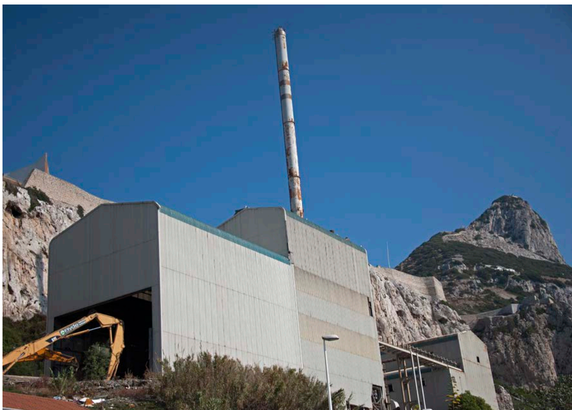
FIGURE Removal of disused incinerator in July 2014. 4.3
