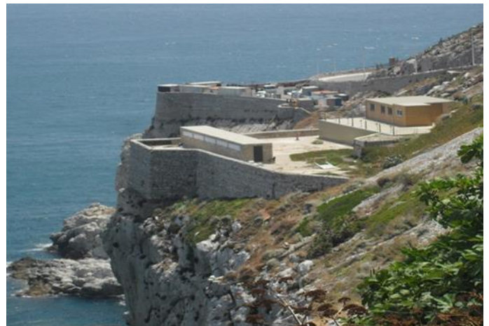
↑Photograph 7: 3 rd Europa Advance Battery from the north after refurbishment in early 2015, with 1 st and 2 nd Batteries to the top.
