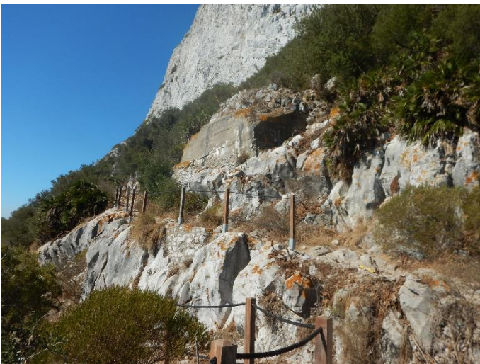
↑General view of the late 19 th -Century Upper Fire Control Structures looking south-east.
