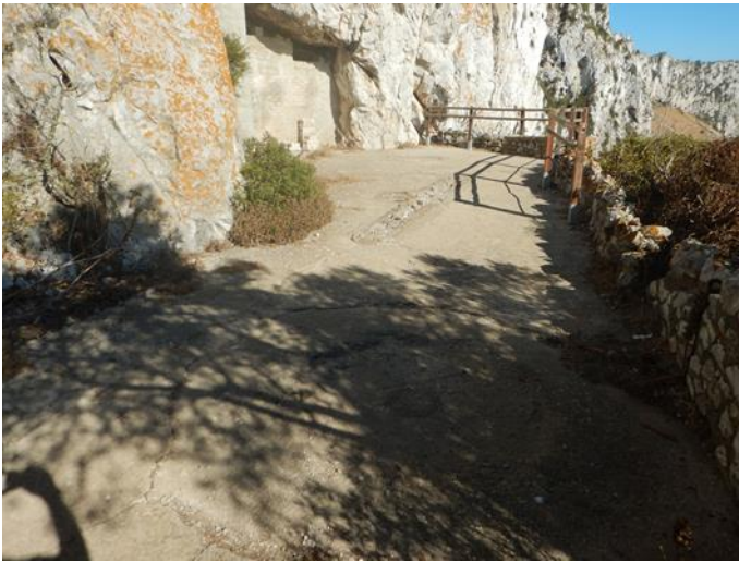
←Gun-mount footings and the north viewing platform. The bricked up caves are on the left of the fenced viewing platform.
