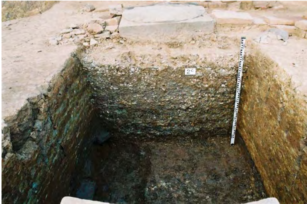
Fig.193: Technique for strengthening a gravel pillar base, Ly Dynasty (11 th -13 th century)
