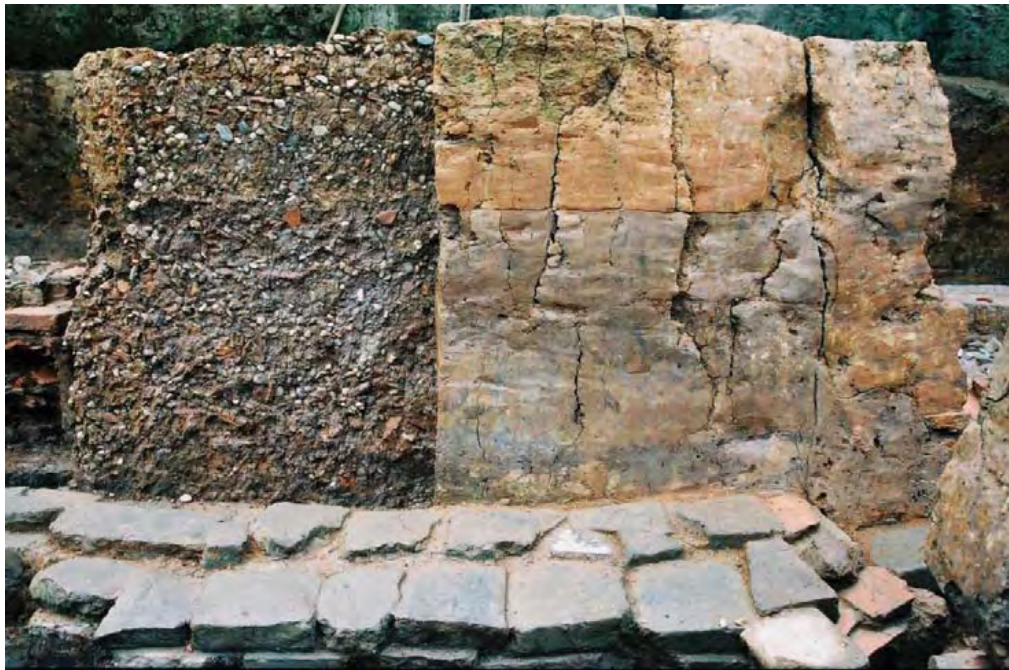
Fig.200: Cross-section of a gravel pillar base , Ly Dynasty (11 th -13 th century)
