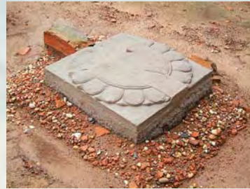
Figure 60: Lotus-flower form stone base for timber column set on a post foundation made of gravel and clay, Ly Dynasty, 11th-12th centuries
