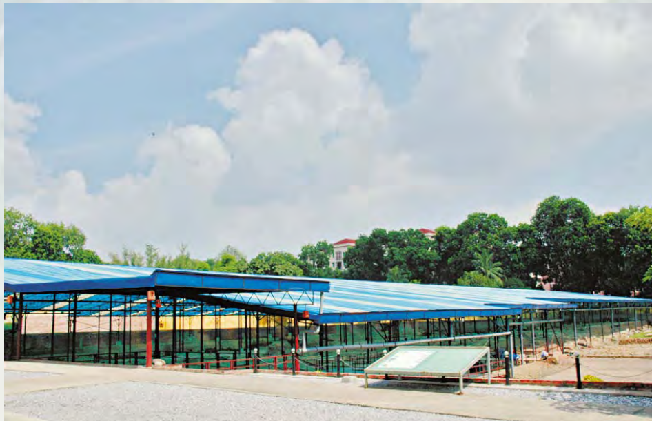
Figures 73-74: Protective roofs for the Archaeological Site at 18 Hoang Dieu Street
