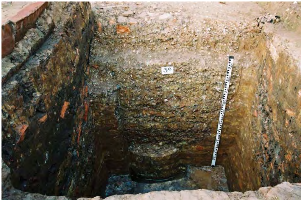
Fig.192: Technique for strengthening a gravel pillar base
