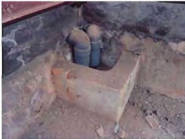
Raccordement cheneau/EP
