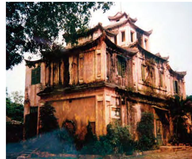
Drawings: section and elevation of Hau Lau pavillon Hau Lau before 1998/2000 restoration — Department of Culture of Hanoi's People's Committee, 1998
