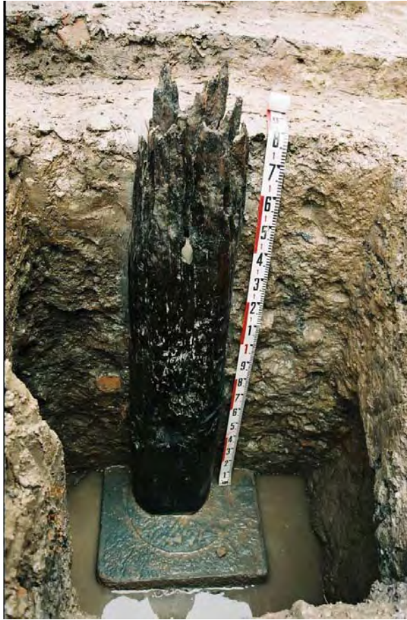
Fig.207: Wooden pillar on a stone pedestal, Ly Dynasty (11 th -13 th century)
