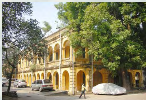
Figure 36: A French style building used for the Operation Department of the Army, Ministry of Defence
