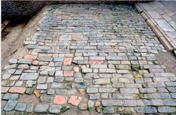
Figure 25: Le Dynasty brick paving.
