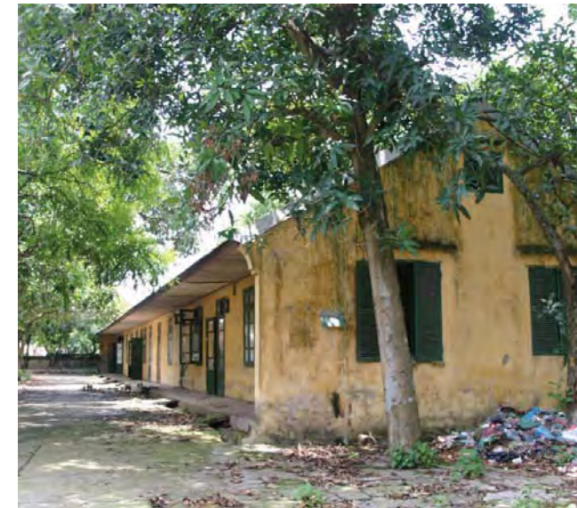
Up: Buildings from first Vietnamese phase Down: Buildings from second Vietnamese phase Photos F. Cristofoli, June 2008
