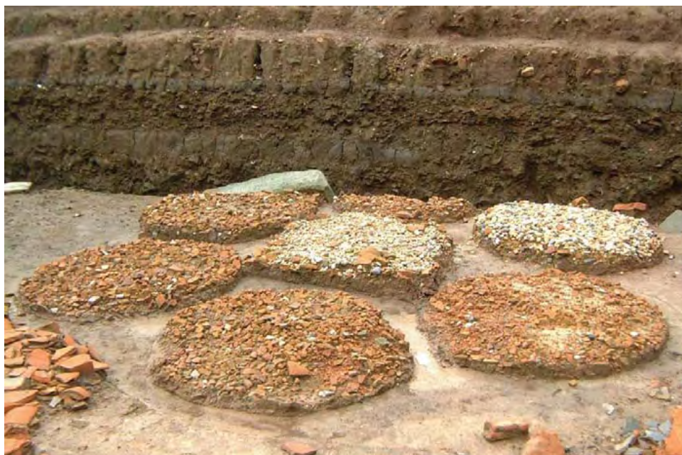
Figure 62: Pillar base made of river gravel and clay of a hexagonal-form building , Ly Dynasty, 11th-12th centuries.
