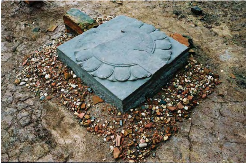
Fig.181: Stone pedestal to support a pillar on the base made of gravels and broken bricks, Ly Dynasty (11 th -13 th century)
