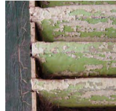
Decayed joinery (insect damage) — Photos S. Ricca, June 2008
