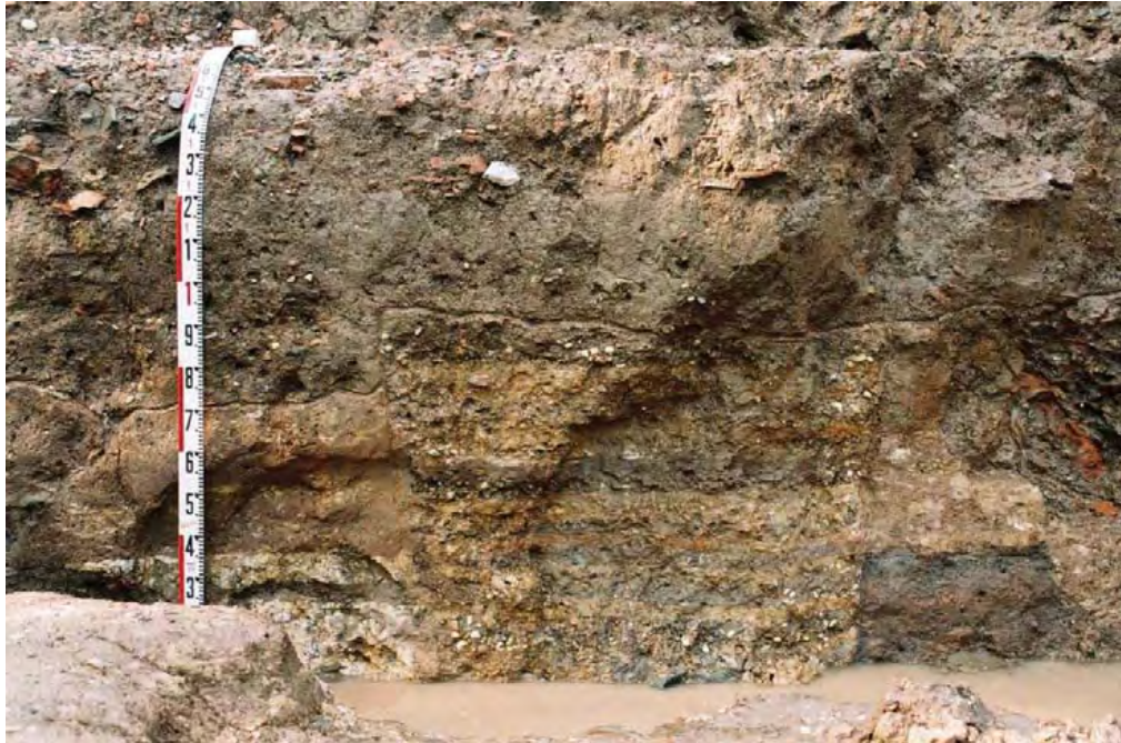
Fig.189: Technique for strengthening a gravel pillar base, Ly Dynasty (11 th -13 th century)
