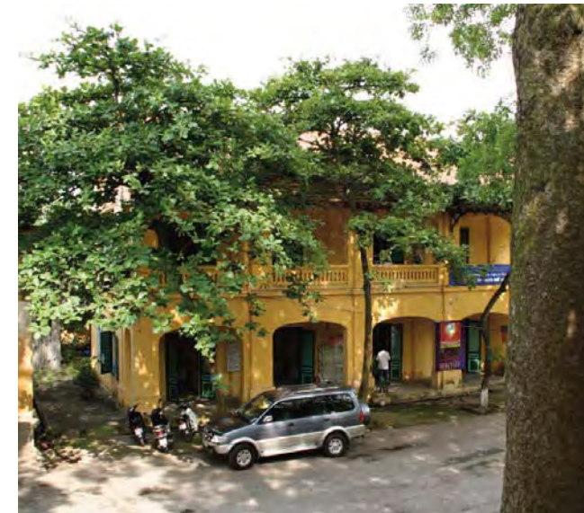
Building N° 33 (French phase) Building N° 19 (French phase) Building N° 16 (French phase) Building N° 24 (French phase) Photos F. Cristofoli, June 2008
