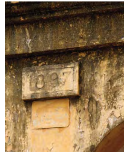
Stratigraphic analysis of the limewash colour Degradation produced by the rusting of a metal beam Limewash deterioration — Photos F. Cristofoli and S. Ricca, June 2008
