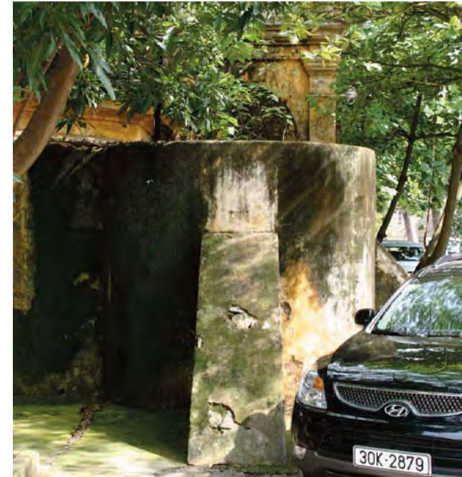
Concrete bunker: external buttress — Photo F. Cristofoli, June 2008
