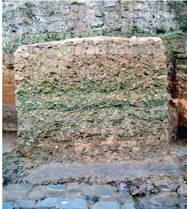
Figure 61: Pillar basemade of river gravel and clay of a building, Ly Dynasty, 11th-12th centuries.
