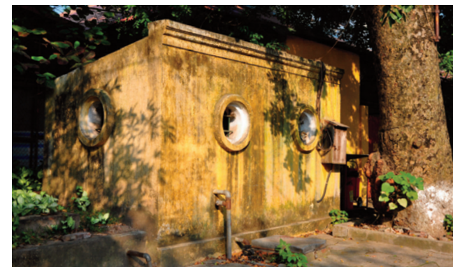
Ph. 38 Station de pompage
