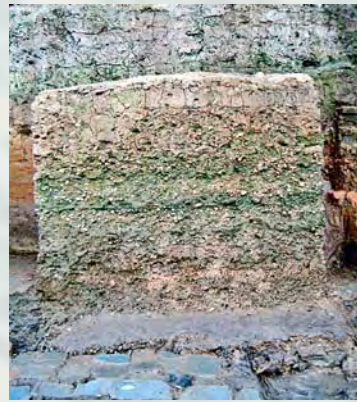
Figure 61: Post foundation made of river gravel and clay, Ly Dynasty, 11th – 12th centuries
