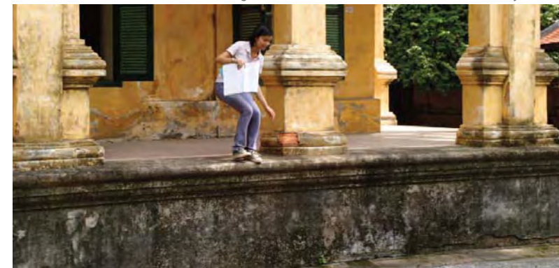
Pediment of building 14 — Photo F. Cristofoli, June 2008
