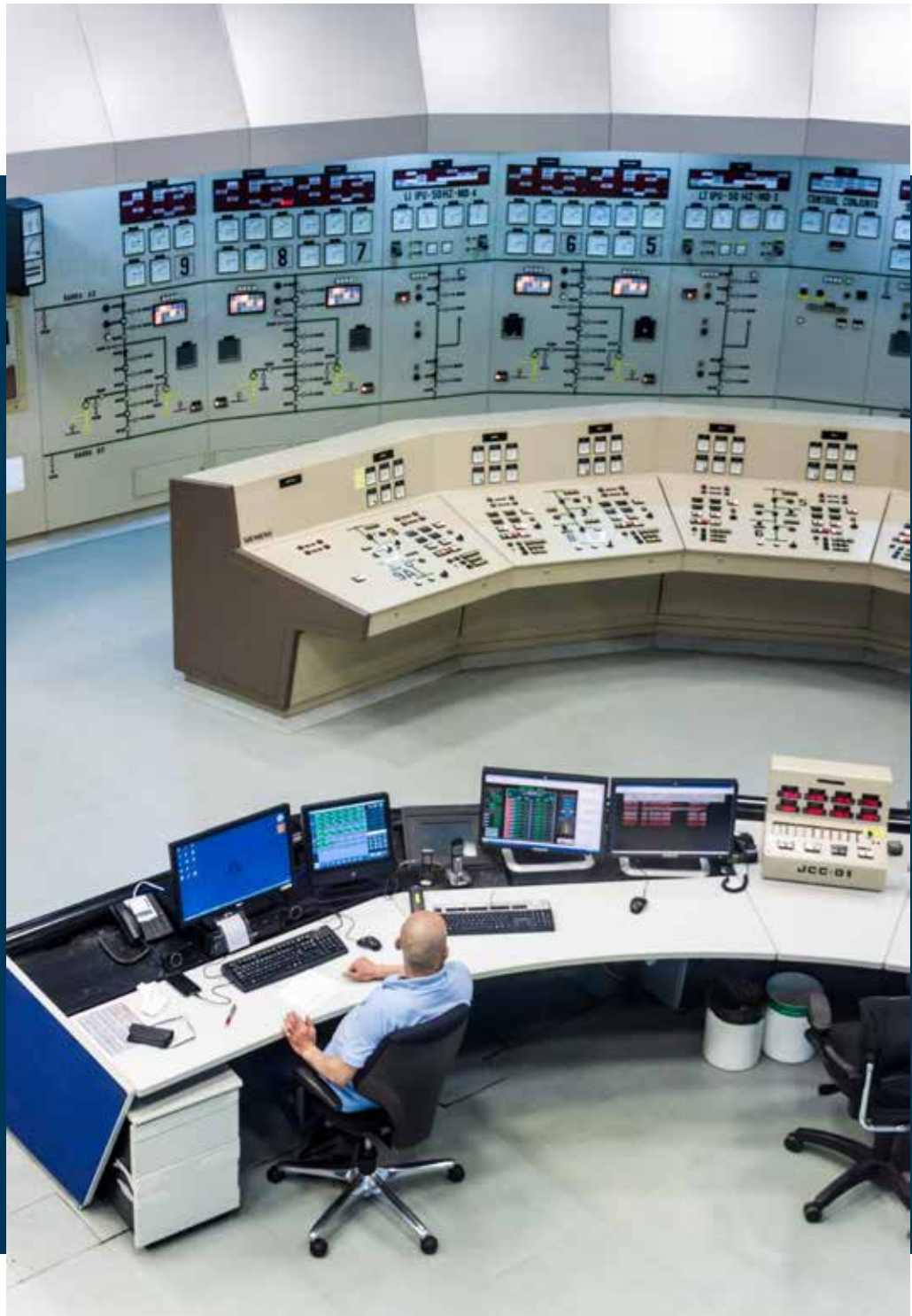
Command room of Itaipu dam on Parana River on the border of Brazil and Paraguay Photo: © Matyas Rehak/Shutterstock.com
