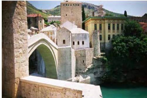
Destroyed in 1993 during the war in Bosnia and Herzegovina, the Old Bridge of Mostar was rebuilt 11 years later. It is a reconciliation symbol. (© A. Roussel/UNESCO)
