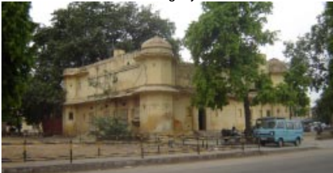
c. The Jaleb Chowk, once an impressive forecourt to the royal palace today represents a picture of neglect and left over space. Random growth of shrubs, broken railings, and buildings in need of repairs mark this chowk.
