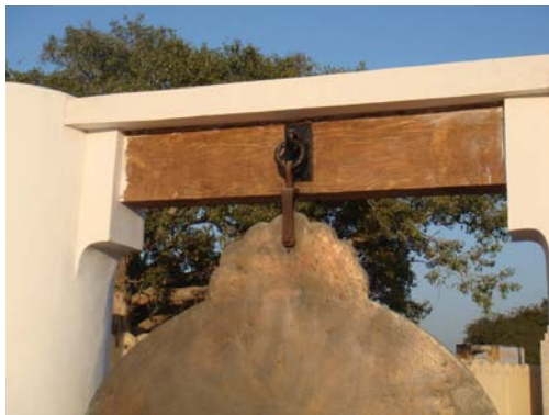
Fig.8: The Yantra Raj with replaced wooden beam
