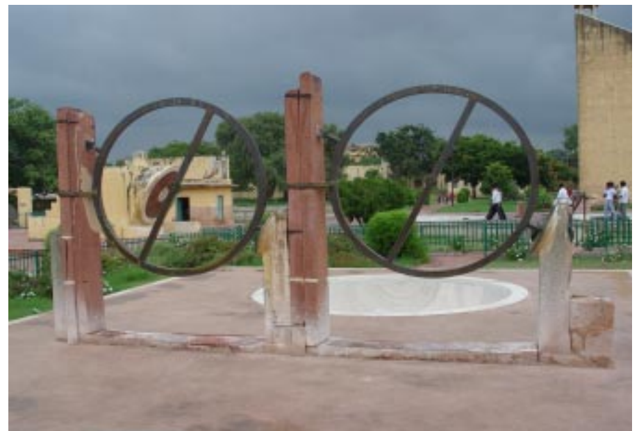
e. Structural damages in Chakra nad Kapali yantra are critical.
