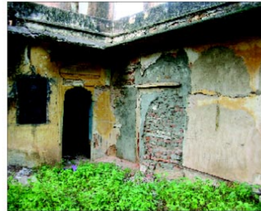
23. ARCHES ARE FILLED UP BY BRICK
