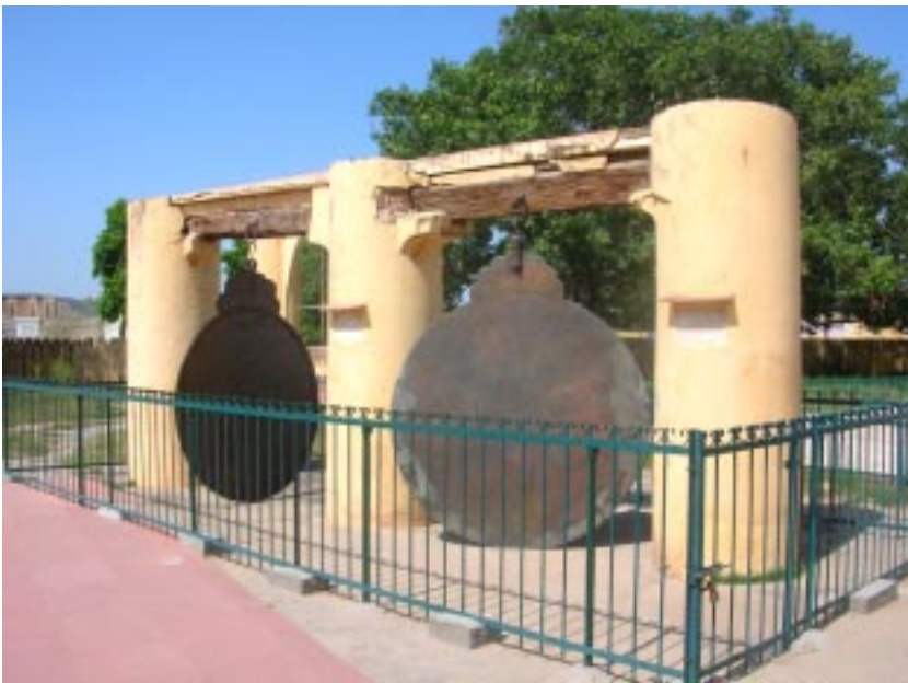
c. Structural damages like cracking of the load bearing timber beams in Yantra Raj.
