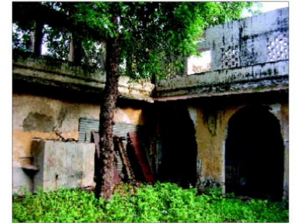
24. ARCHES ARE FILLED UP BY BRICK
