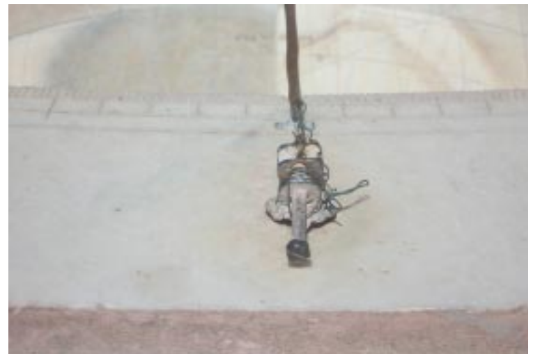
e. The cables which mark the azimuth in the Great Jai Prakash Yantra have been fixed with poor details.
