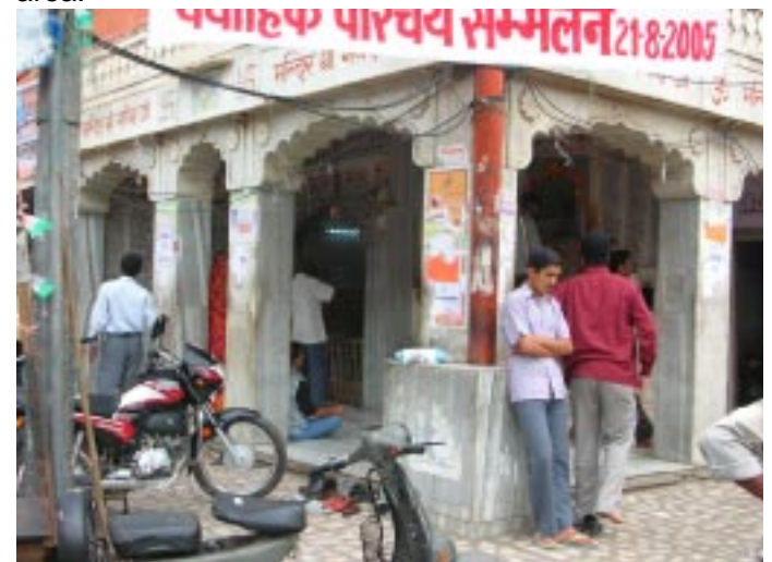
c. Random hoardings in terms of size, font, material, colour, exposed electrical lines, unorganised parking all contribute towards the chaos that one experiences in the area.
