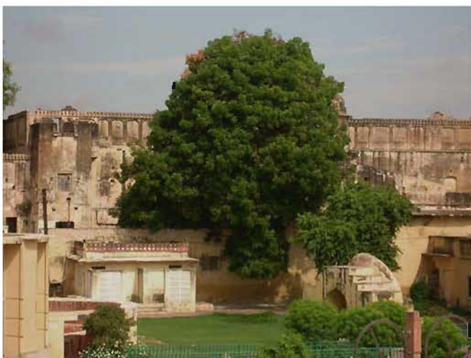
View of toilet block
