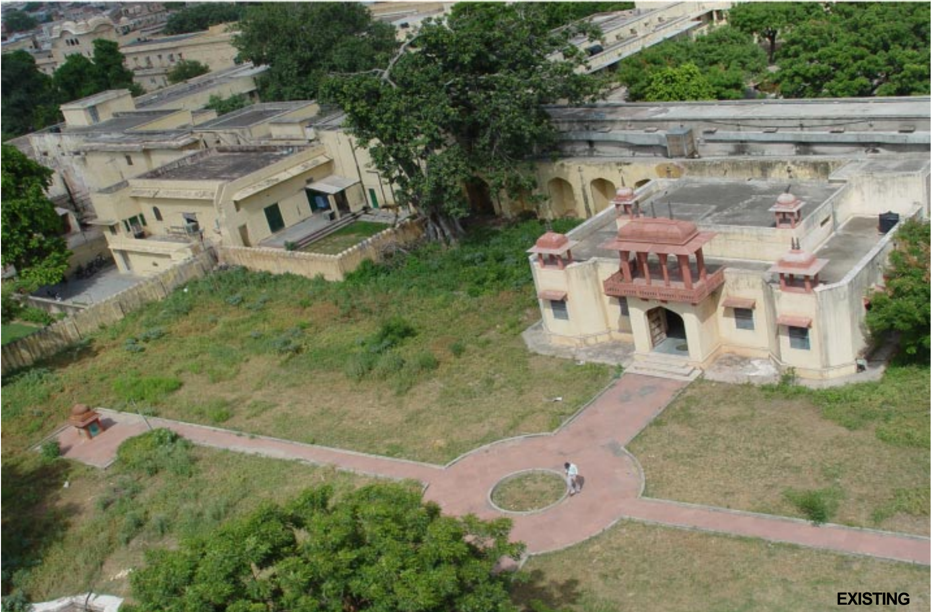
The corner of the site is encroached upon by the police offices. The new building built in the complex is incongruous with the architectural language of the complex.
