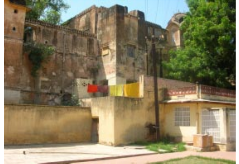
c. Toilet block on site, with an electric pole. Priests hang clothes in devasthan property which overlooks the complex. These elements disturb the historicity of the complex and need to be removed.
