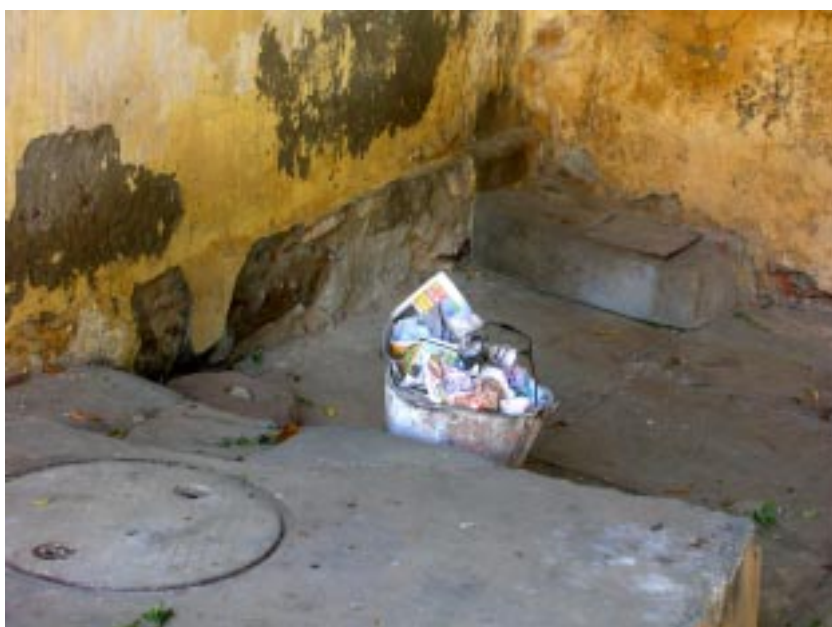
b. The kind of dustbins for collecting garbage leaves a lot to be desired.
