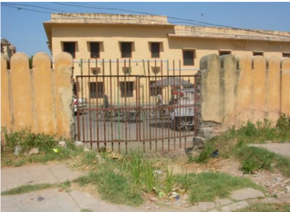
a,b. Movement within the monument has been in a state of flux. Some remnants from earlier attempts of entry and movement.
