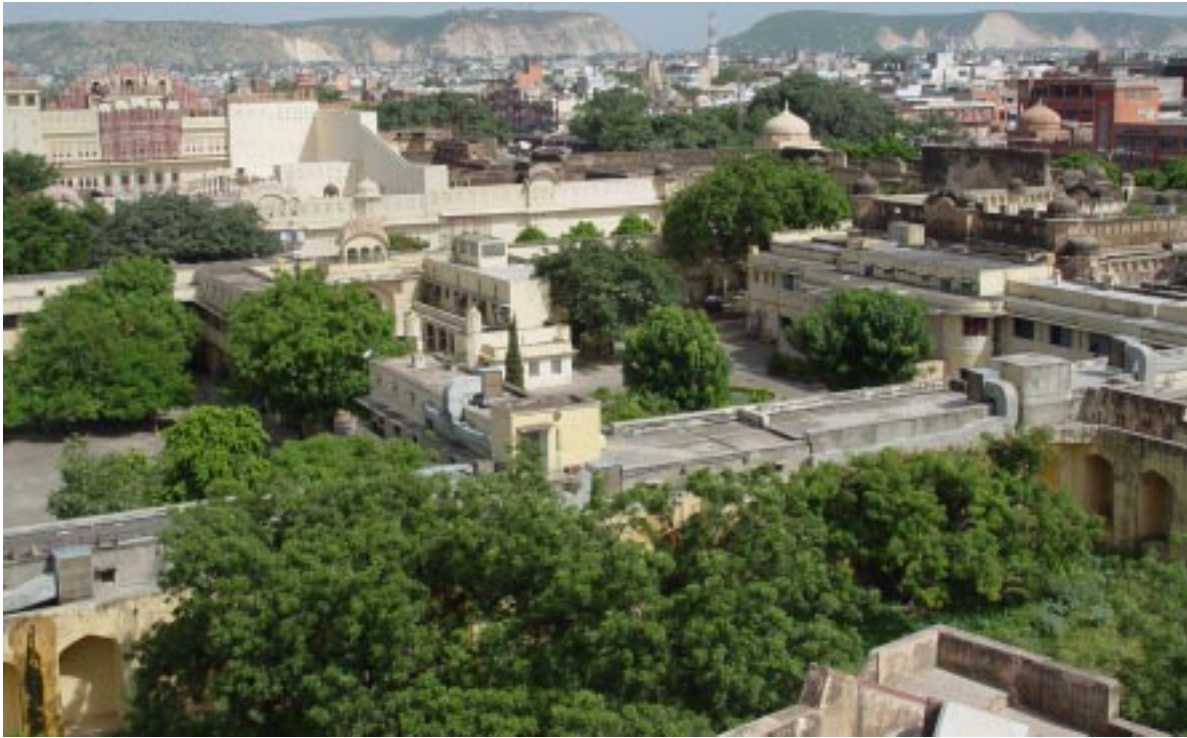
a. The Police Headquarter building with its large courtyard lies between the Jantar Mantar and the Hawa Mahal. This used to be a stable for the palace. Its present function is not congruous to the character of the area. It can become the connection between the two monuments
