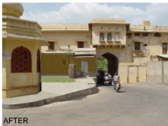
Gate after removing toilets, hoardings and electric boxes
