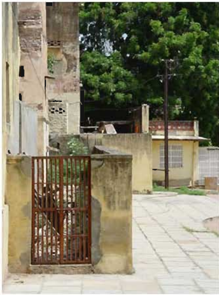
View of dump yard
