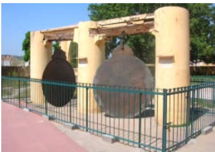
c. Structural damages like cracking of the loadbearing timber beams in Yantra Raja.
