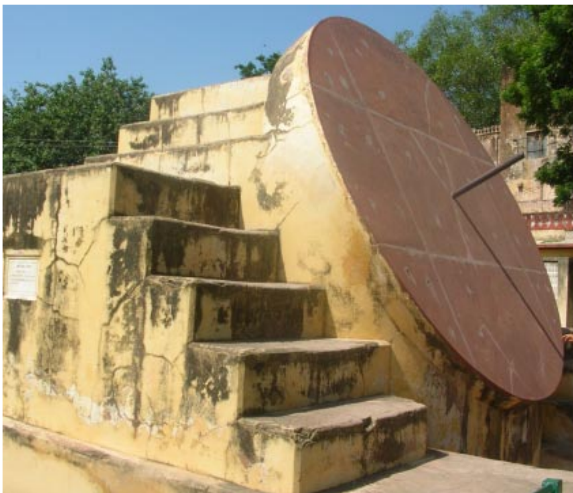
c. The nosing of the stairs is most vulnerable to the movement of the people. They have worn away at most places.
