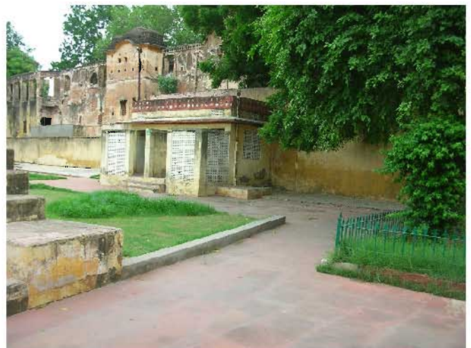
View of toilet block
