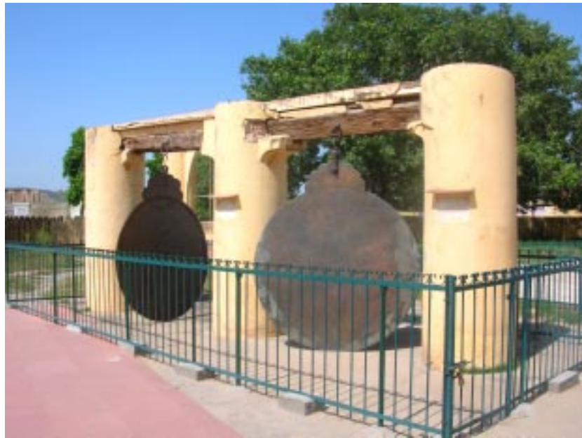
c. Structural damages like cracking of the load bearing timber beams in Yantra Raj.
