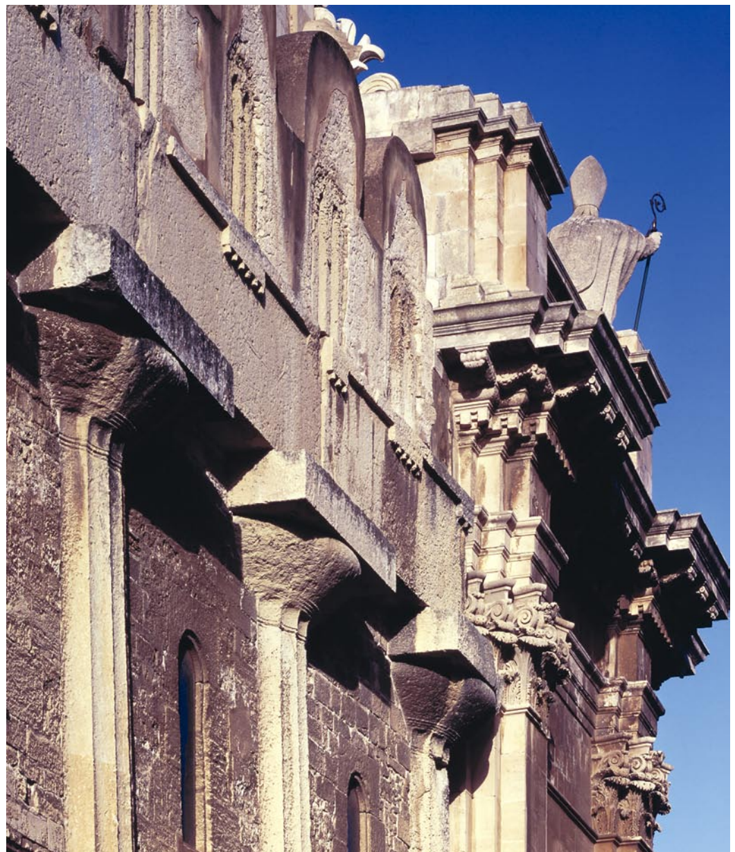
Syracuse Cathedral - Details of the northern facade
