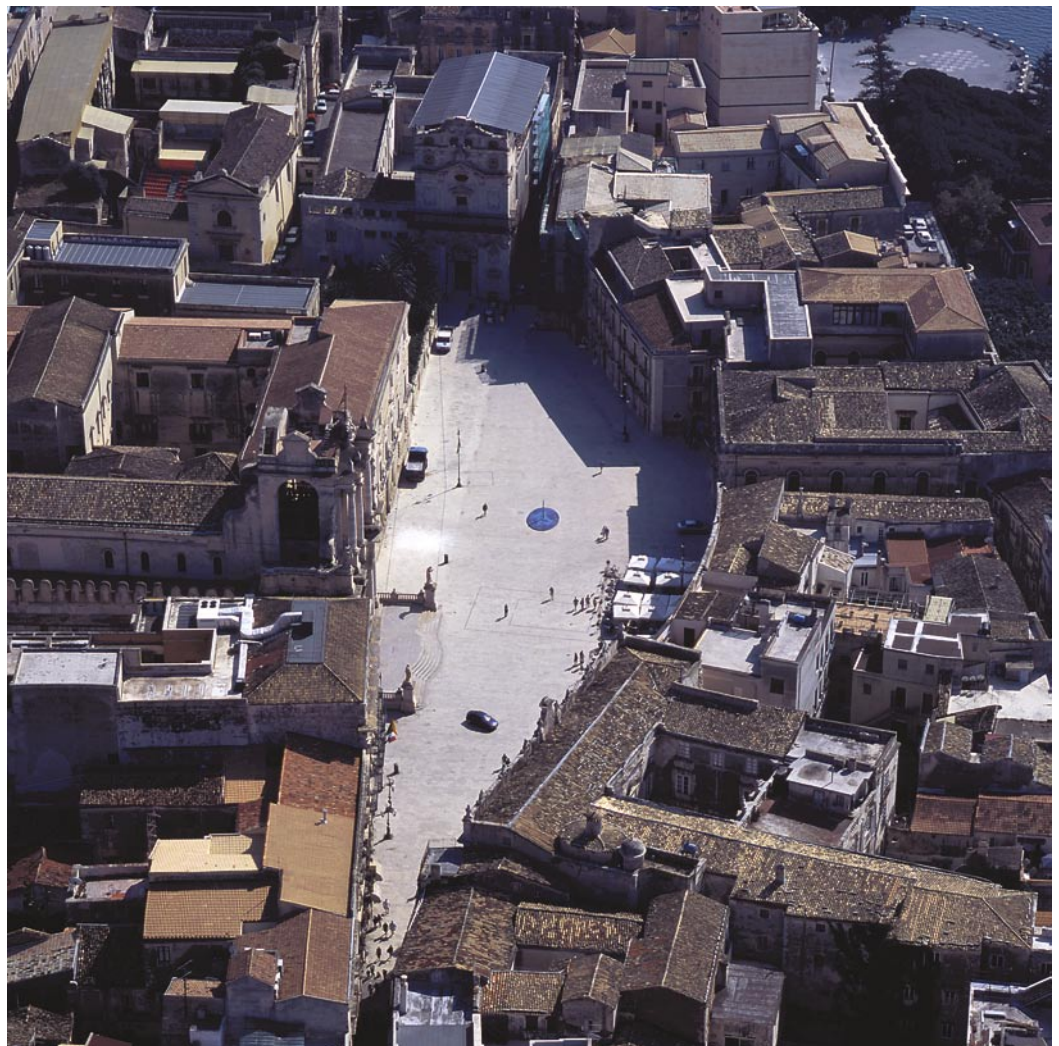
Syracuse Aerial view of Cathedral Square
