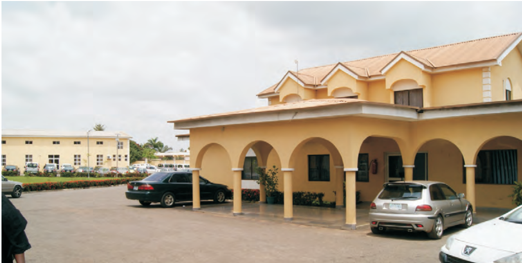
• Centre Administrative Building with multipurpose Auditorium in the Background
