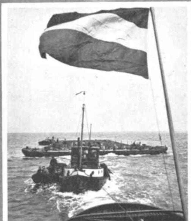
A dike in the making. From an artificial island (top photo) ribbonlike form of dike begins to wind its way across what was once Zuider Zee. When tugs and workers have completed their task and pumped out water, the dike will protect a new polder, and the Netherlands will have won more productive land from the sea.
