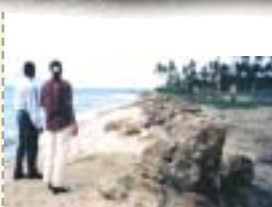
Planning officials inspecting a newly constructed rock revetment at Pinney's Cotton Ground, 1999
