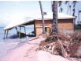
This restaurant at Pinneys Beach was 30 metres from the sea when it was opened in August 1995. One month later it was destroyed by Hurricane Luis. The greater the distance from the sea, the safer the building
