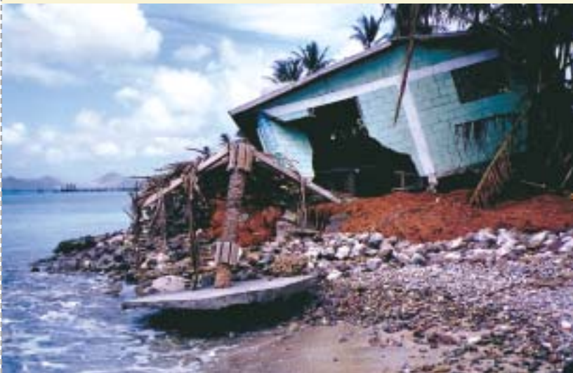
Damaged beach bar at Golden Rock, Pinney's Beach, after Hurricane Luis, 1995
