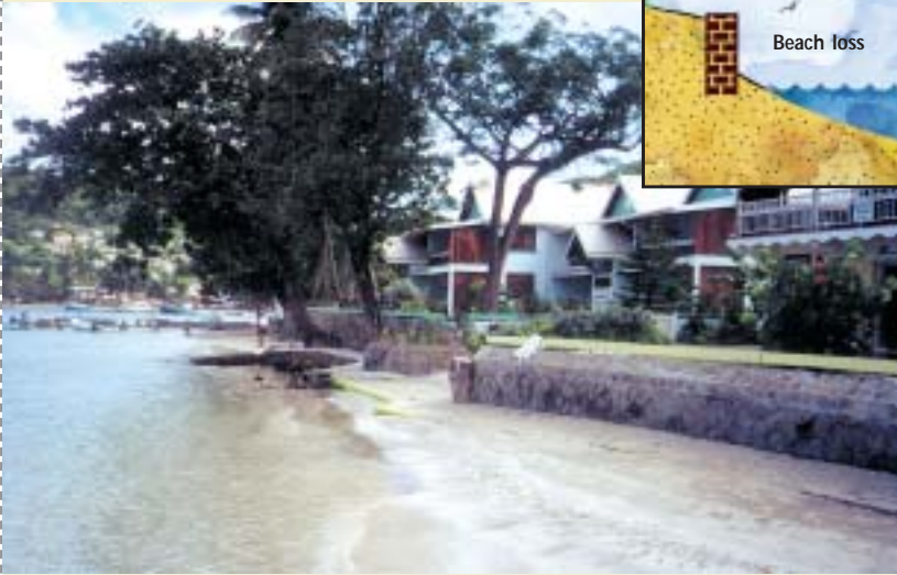
Retaining wall at Port Elizabeth, Bequia, 2000
