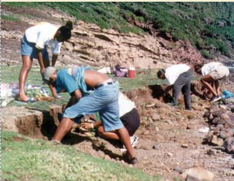
Students building stone barriers and planting cacti to prevent soil erosion, Park Bay, Bequia, 1997
