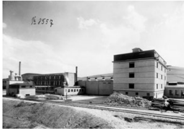
Fig. 18: Entire property from the north-east, 1 st building section (1912)
