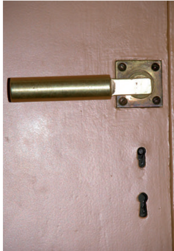
Fig. 93: Main building, main staircase, 1 st floor, door detail (2002)
