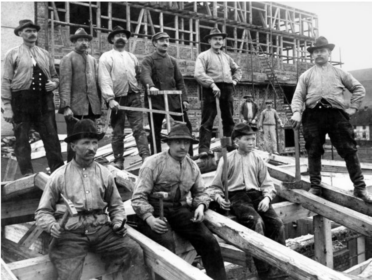
Fig. 19: Extension of the store house, carpenters (1913/14)
