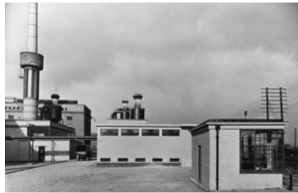
Fig. 48: Rail-lifting jack/rail-car scales, chip and coal bunker, engine house, smoke stack, storehouse, view from the south, photo by Edmund Lill (1924)
