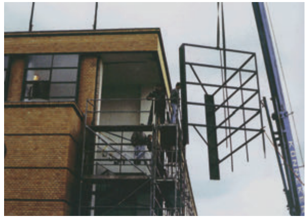
Fig. 73: Main building, refitting of window elements (1989)
