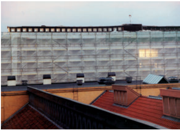
Fig. 72: Storehouse during restoration (1999)
