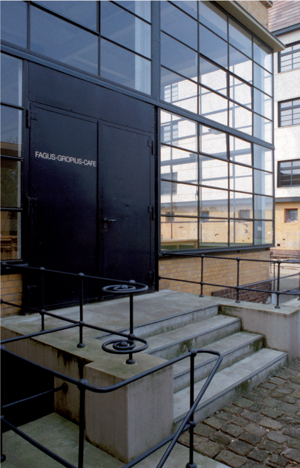
Fig. 81: Engine house, entrance (2002)
