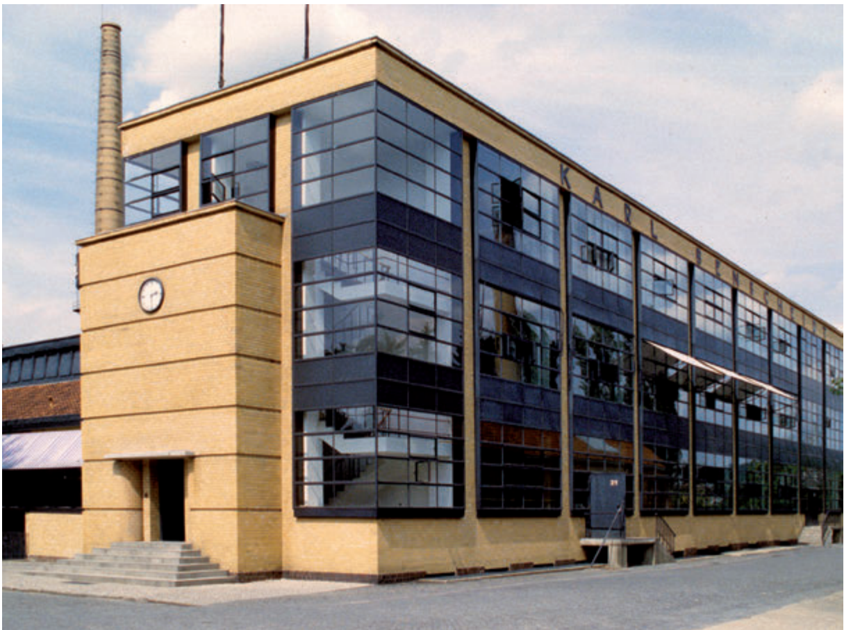
Fig. 32: Main building viewed from the south-west (2002)
