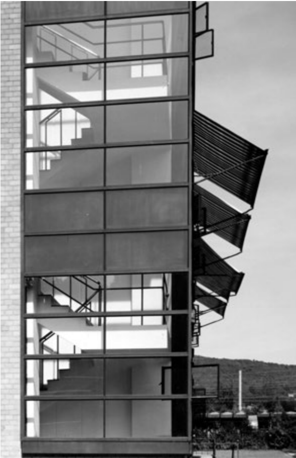
Fig. 33: Main stairway, paned corner, view from the west (1999)
