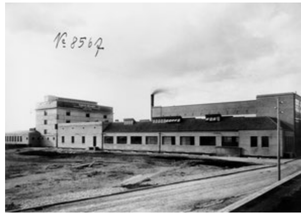
Fig. 67: Entire property from the south-west, 1 st building section (1912)
