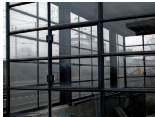
Fig. 51: Rail-lifting jack, rail-car scales, railway side, window front (2002)
