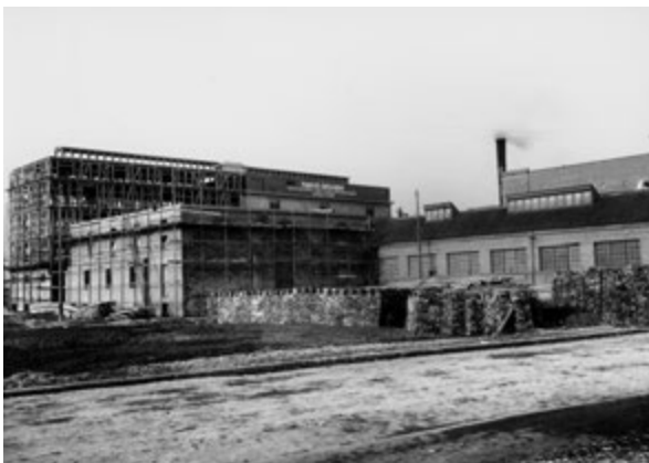
Fig. 20: Extension of the drying house and store house, 2 nd building section (1913/14)
