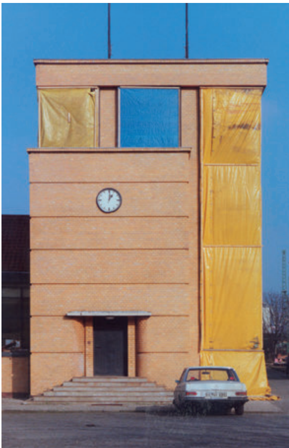
Fig. 74: Main building during the restoration (1987)
