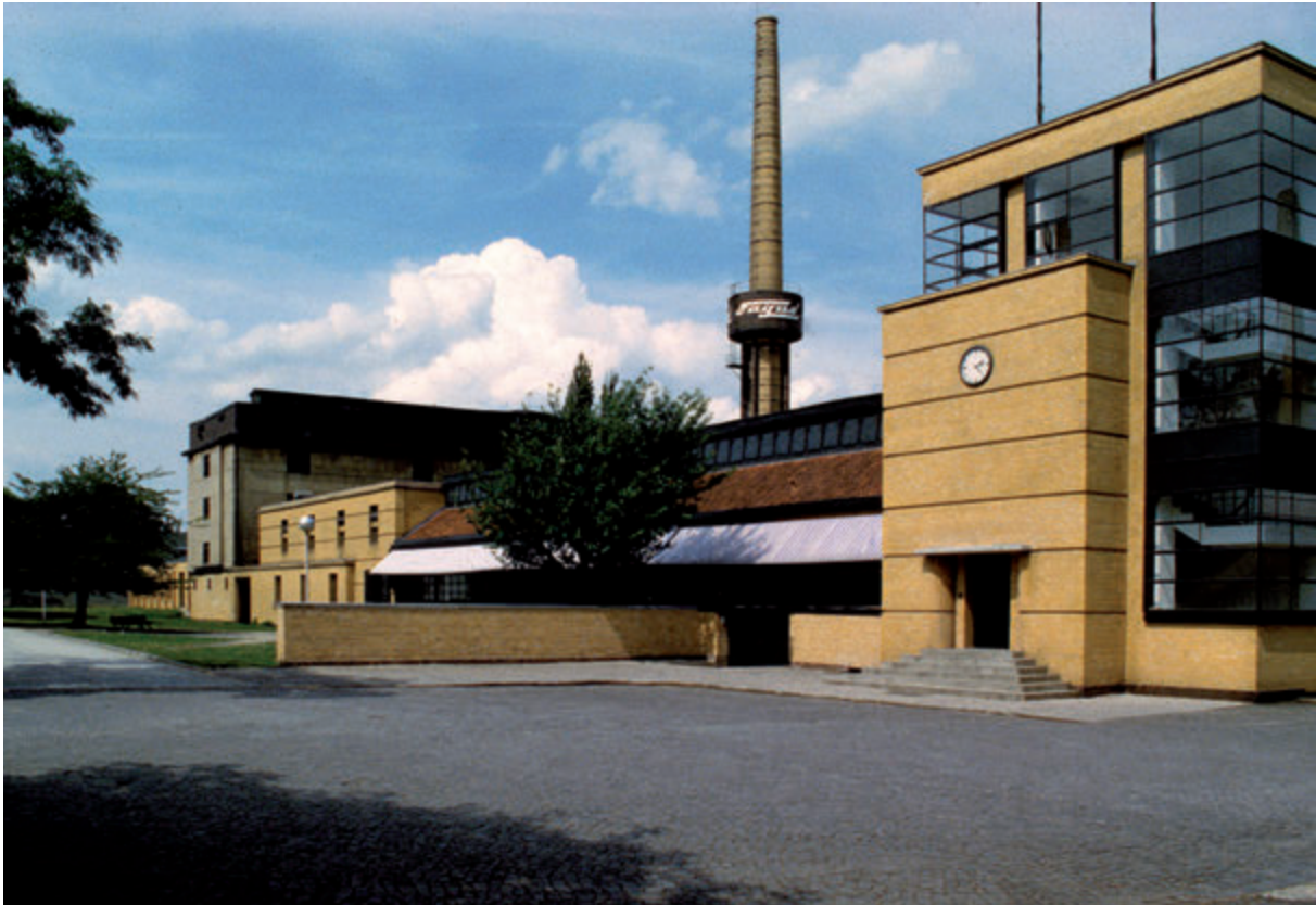
Fig. 22: South-western view with main building, workroom, drying house and store house (2002)
