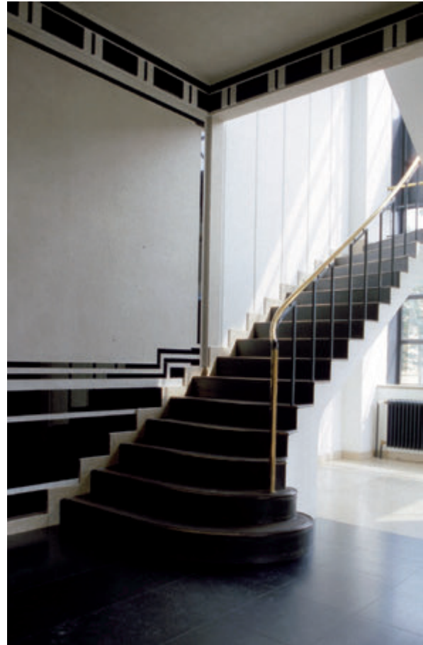
Fig. 38: Main building, foyer, staircase (2002)
