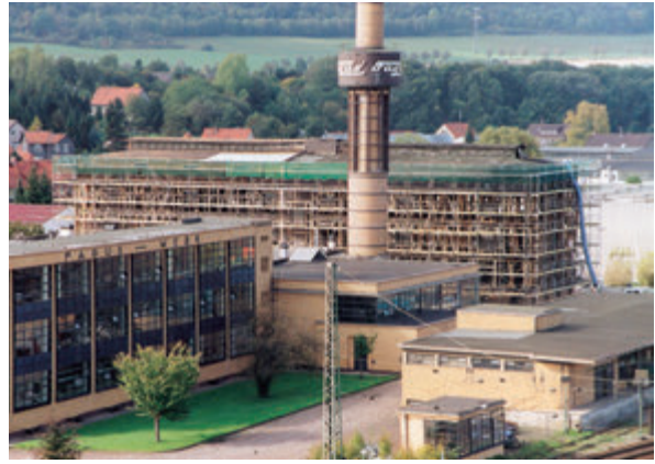
Fig. 71: Storehouse during restoration (1999)
