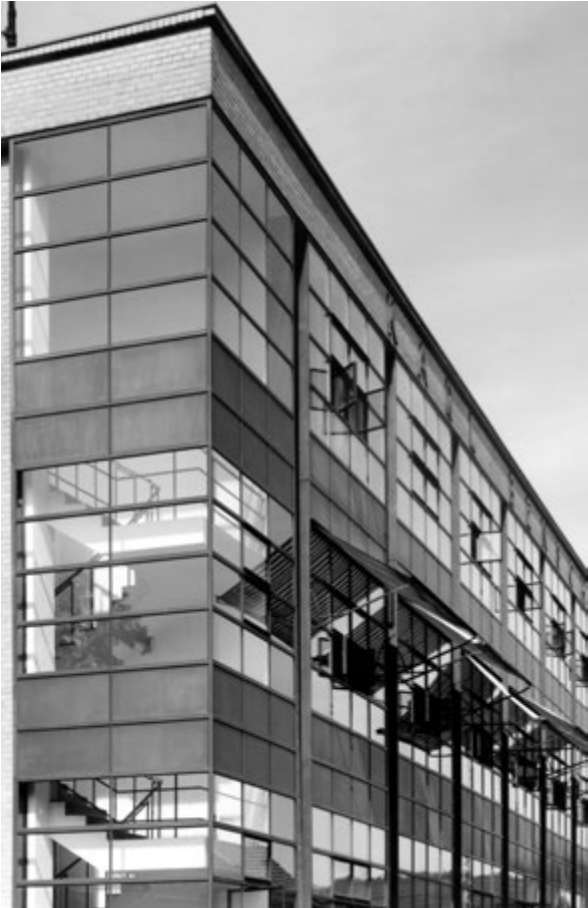
Fig. 35: Main building, view from the south-west (1999)
