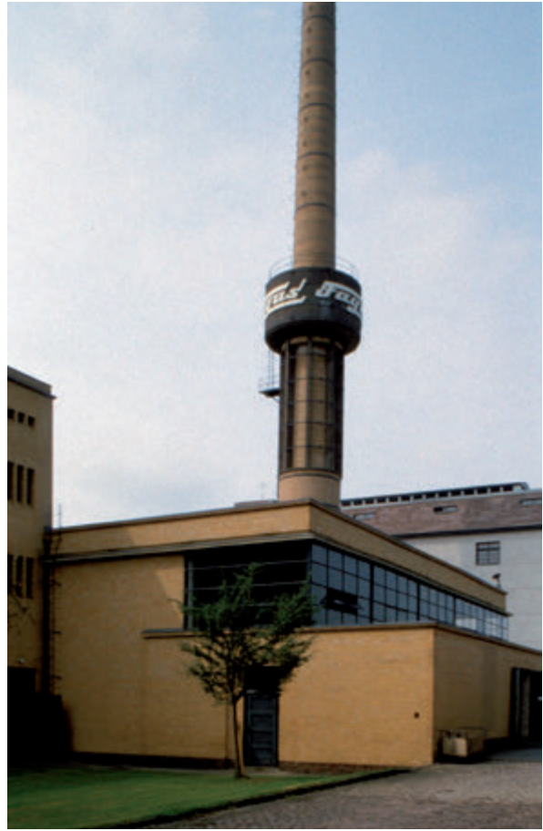
Fig. 44: Engine house, smoke stack, store house, view from the south-east (2002)
