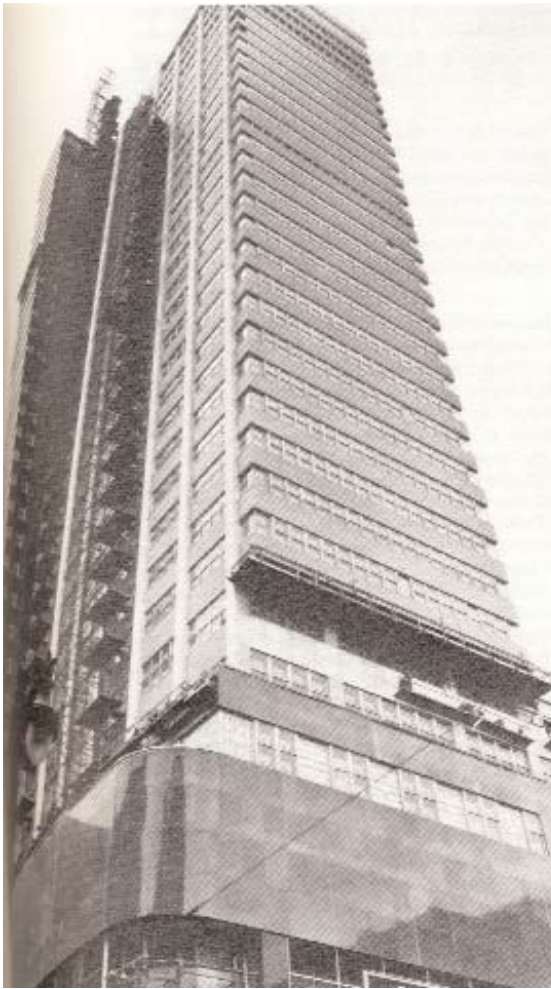
34 Philadelphia Savings Fund Society Building, Philadelphia, USA, 1929 by George Howe and William Lescaze
