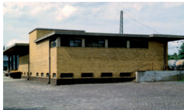
Fig. 49: Chip and coal bunker, view from the south-west (2002)
