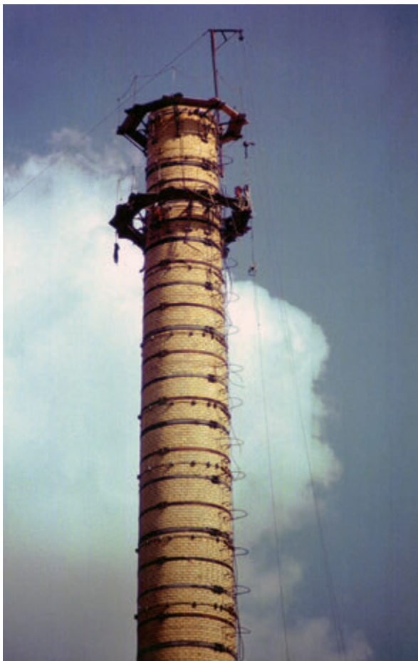
Fig. 47: Smoke stack, brickwork renovation (1988)
