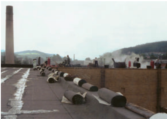
Fig. 77: Main building, roof renovation (1985)
