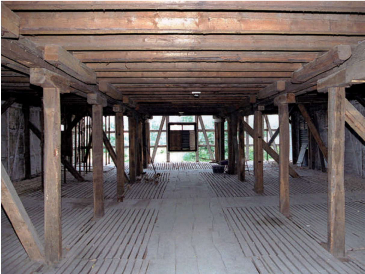
Fig. 112: Storehouse during renovation (1998)
