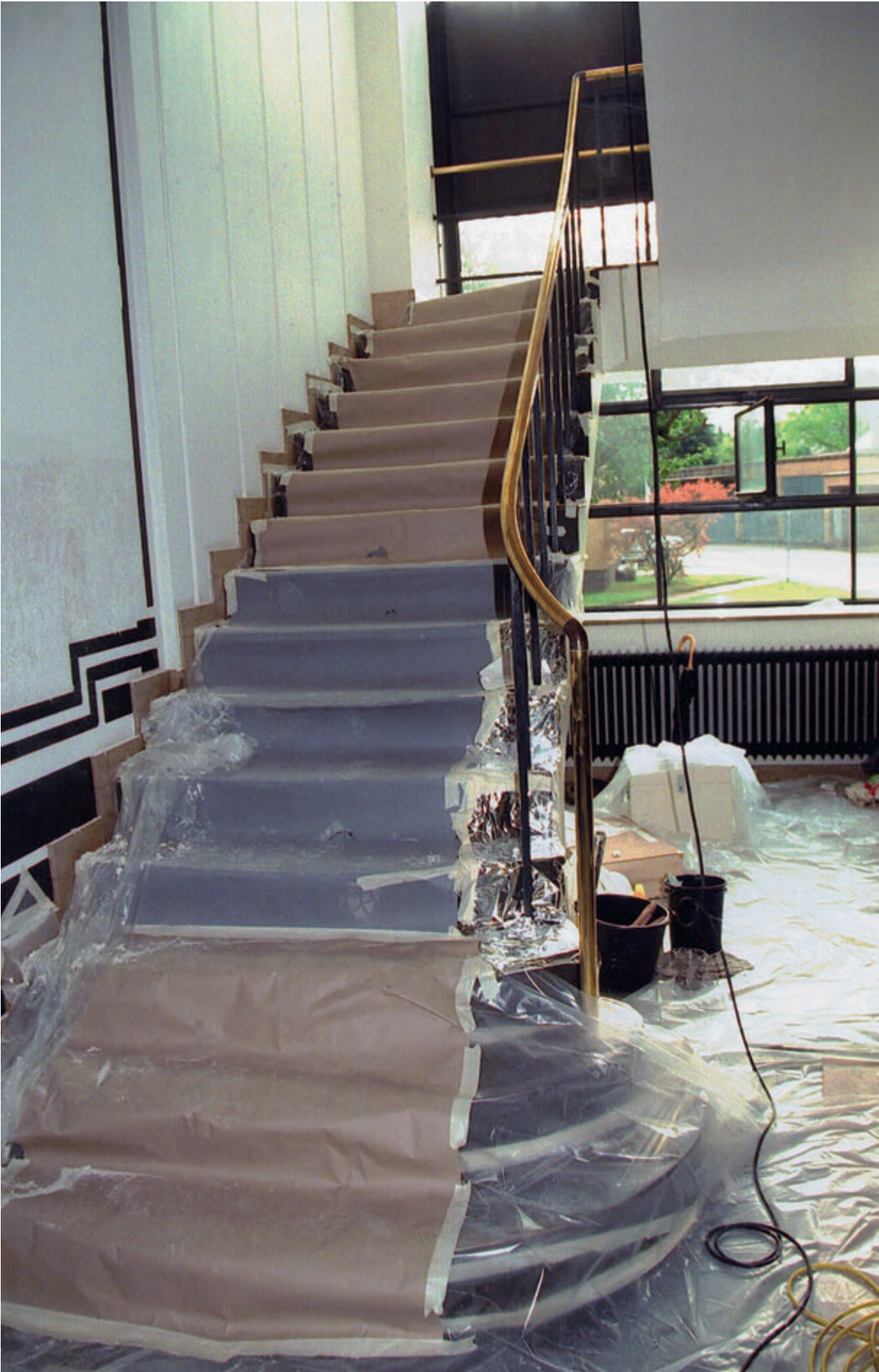
Fig. 111: Main building, restoration of the main staircase (1995)
