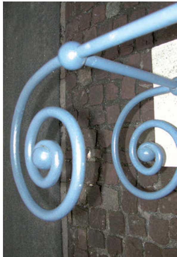
Fig. 91: Engine house, gas pipe railing (2002)
