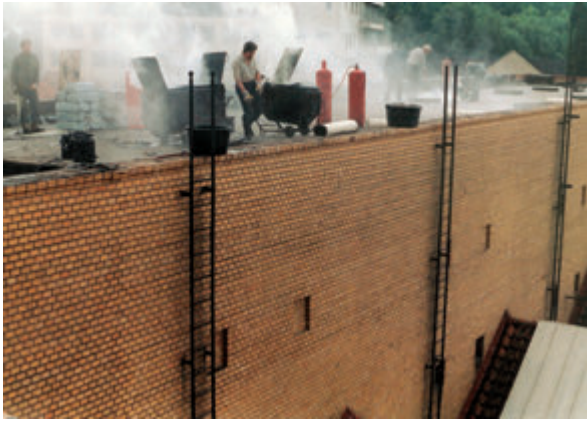
Fig. 70: Main building, roof renovation (1985)
