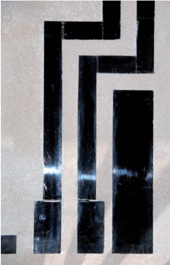
Fig. 37: Main building, foyer, detail of opal glass bands (2002)
