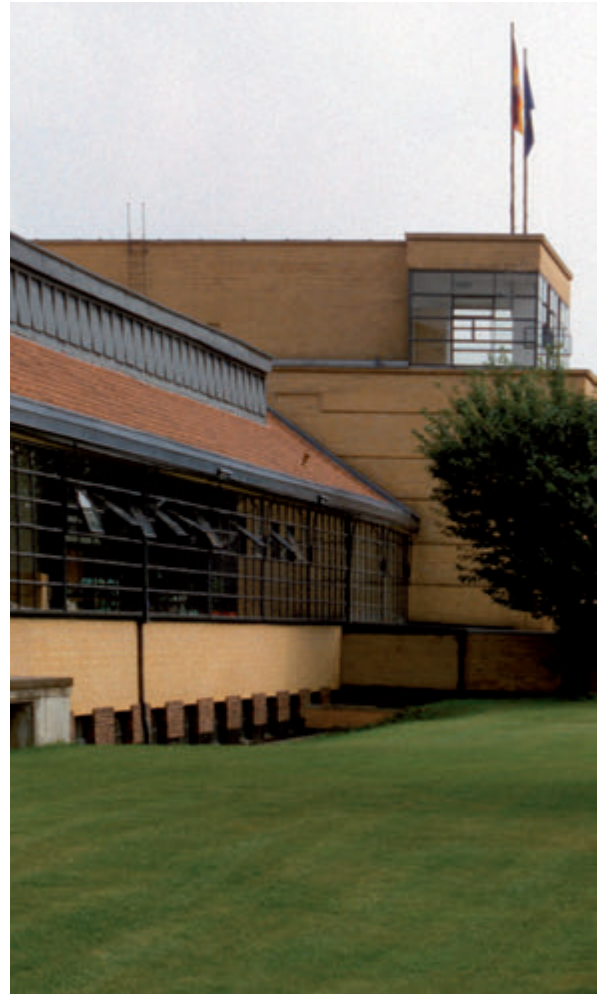
Fig. 26: View of the workroom and main building from the north-west (2002)
