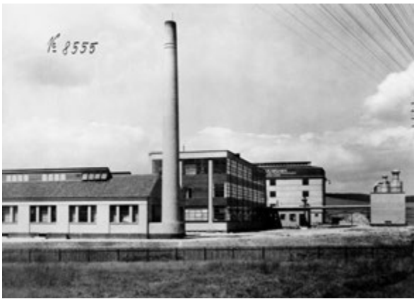
Fig. 66: Entire property from the south, 1 st building section (1912)
