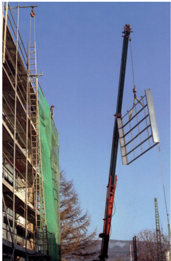
Fig. 75: Main building, refitting of window elements (1989)
