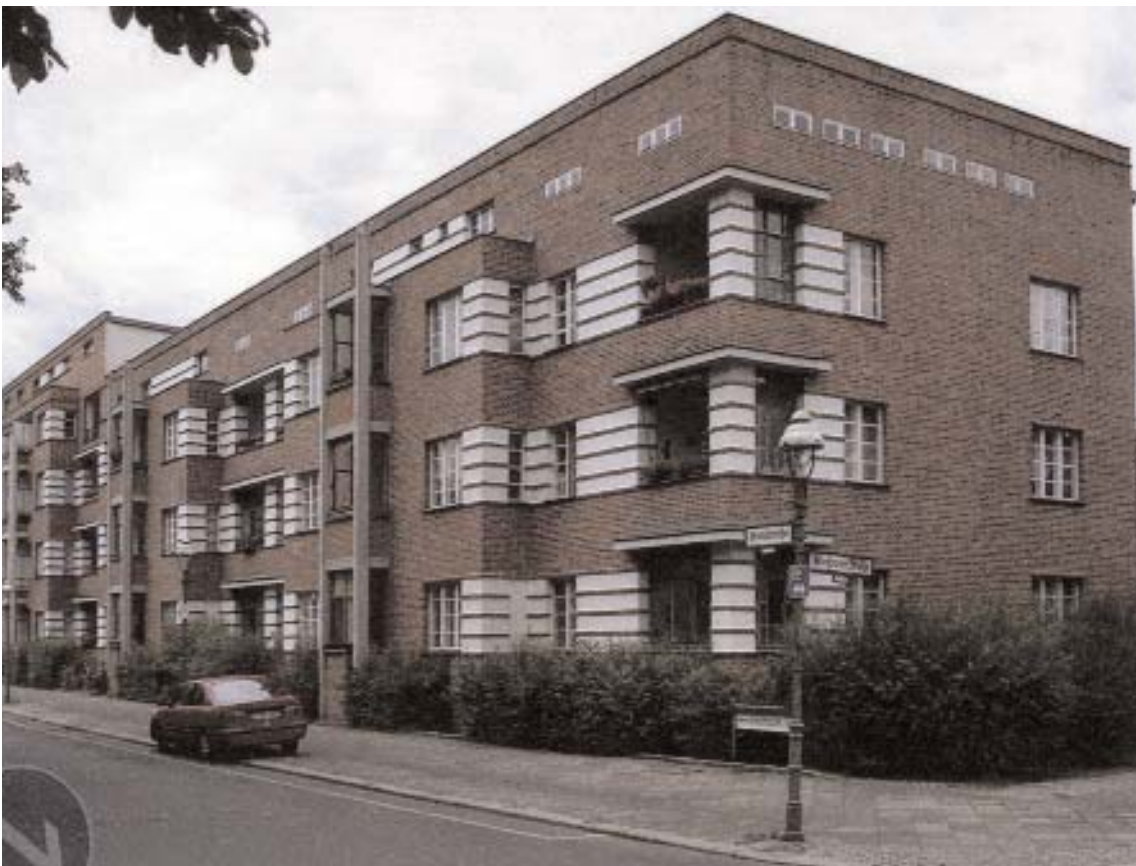
4 Berlin Modernism Housing Estates, Berlin, Germany, 1919-1931 by Bruno Taut, Otto Bartning, Hans Scharoun, Walter Gropius et al
