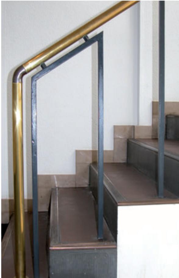
Fig. 41: Main building, staircase, hand rail 1 st floor (2002)
