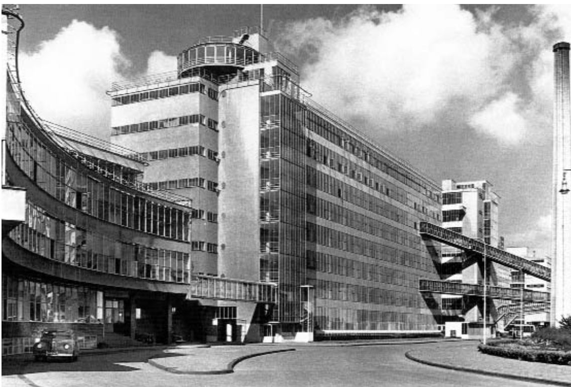
25 Van Nelle factory, Rotterdam, Netherlands, 1926-1930 by Leendert van der Vlugt and Andreas Brinkman
