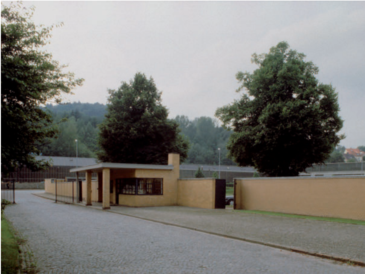
Fig. 60: Entrance with gatekeeper's house, view from the south-east (2002)
