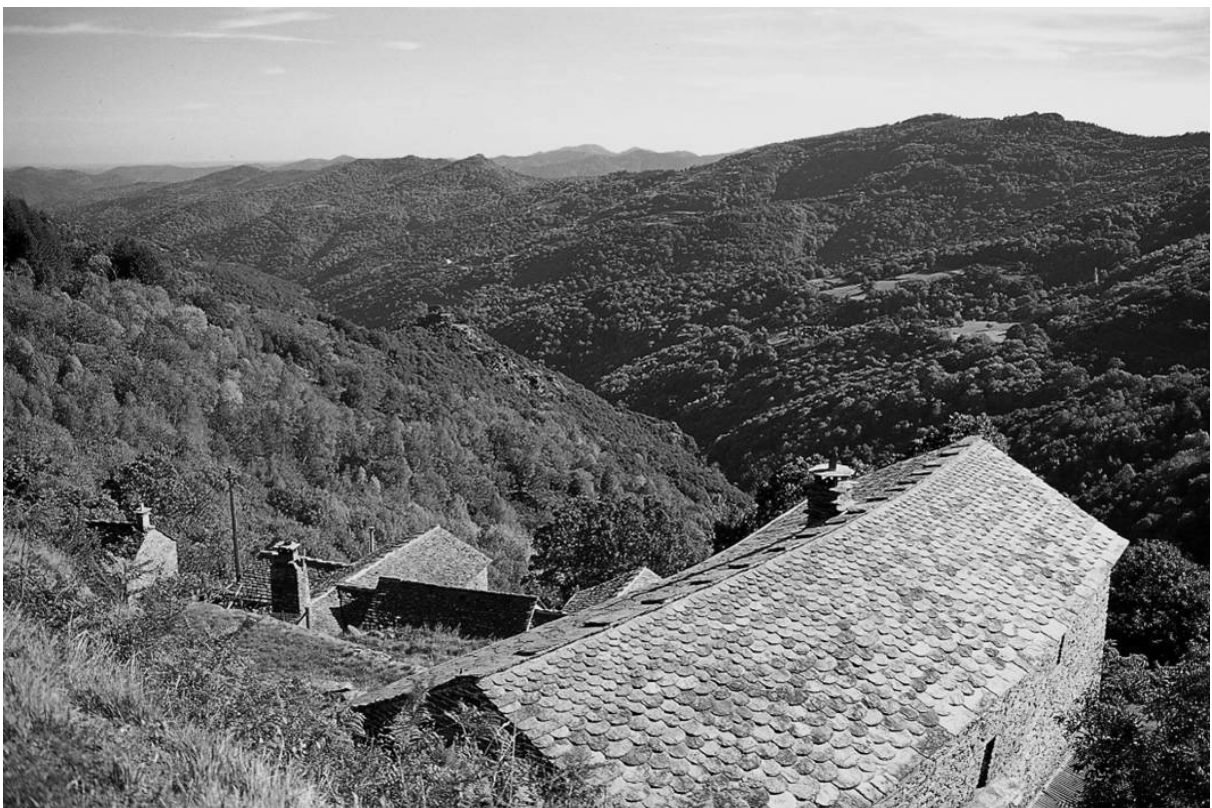
Roof of shell-shaped slates
