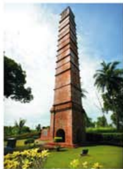
The restored Chimney (2018)
