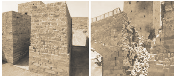
Marid Old Dam before and after image. Photo credit: Hussain Bukhaiti. Satellite imagery collected on 29 October 2015 shows one of the retention towers severely damaged with visible debris in the middle section of the Southern Dam sluice.
