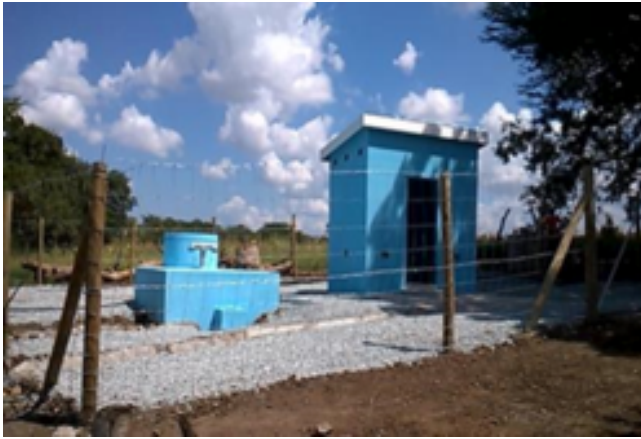
Pumping water out of a sand dam (Swaziland) Photo: Department of Water Affairs (2015).
