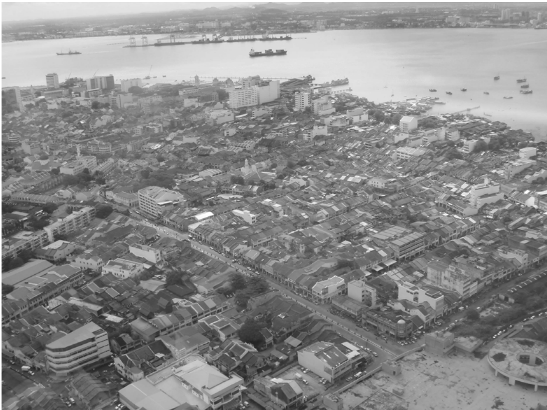
Aerial view of the historic city
