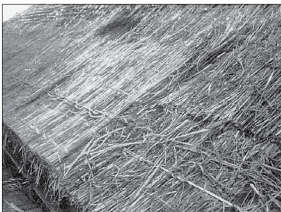
5 軒付け(水切茅) Thatching of eaves
