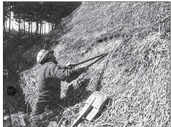
6 刈り上げ Cutting of the surface
