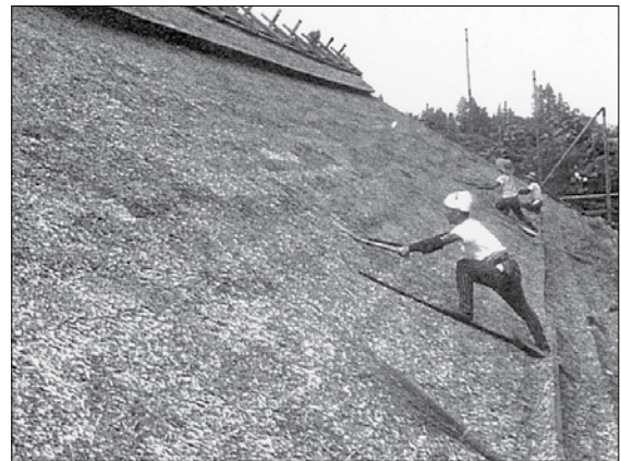
10 屋根面刈込み(ハサミ) Cutting of roof
