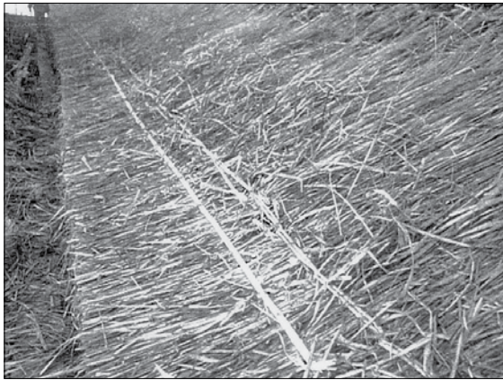
7 軒付け完了 Completion of eaves
