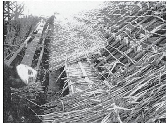
2 軒付け(山茅) Thatching of eaves
