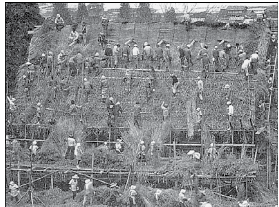
6 平葺き Thatching of field
