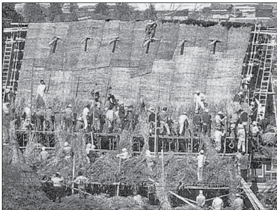
5 軒付け Thatching of eaves
