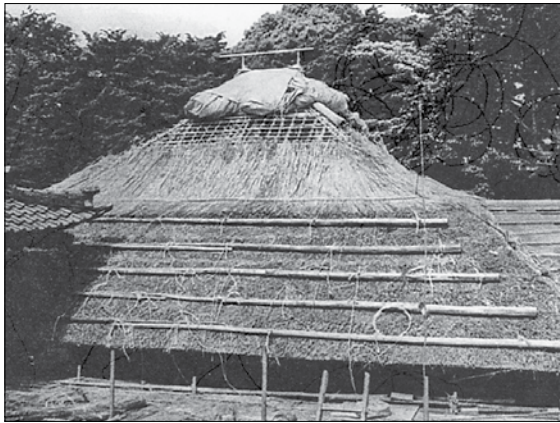
7 茅葺き上げ中 Thatching of field
