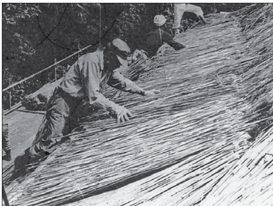
5 平葺き Thatching of field
