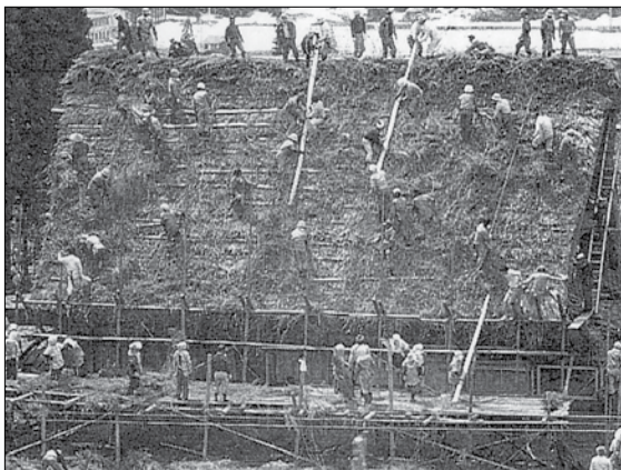
7 棟包み Thatching of ridge
