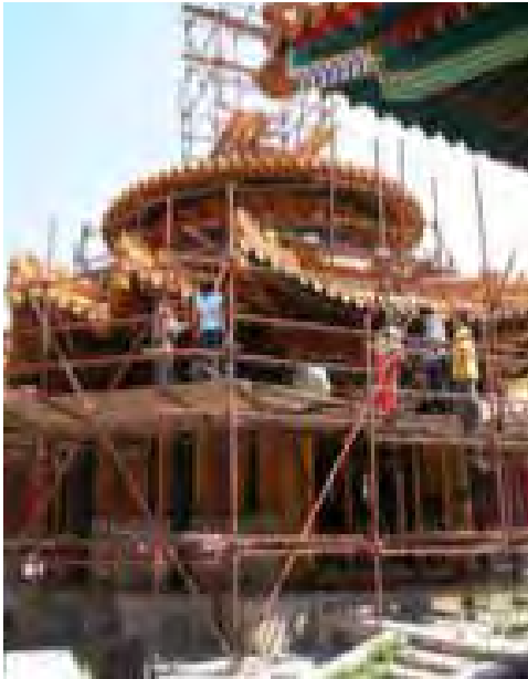
Pic 14: The restoration of Xiangyun Pavilion
