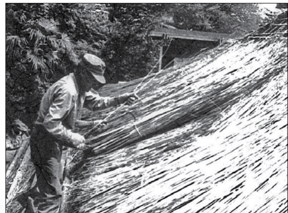
6 平葺き Thatching of field
