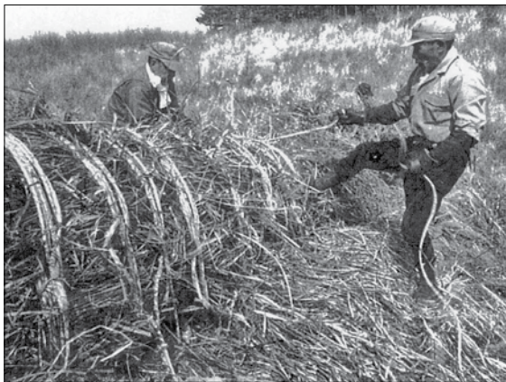
5 棟造り(シタマル Thatching of ridge
