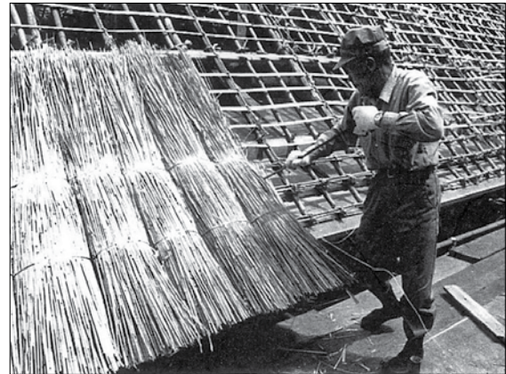
2 軒付け(ヨシ) Thatching of eaves
