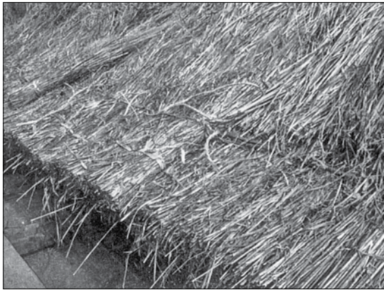
3 軒付け工程(水切り茅 Thatching of eaves
