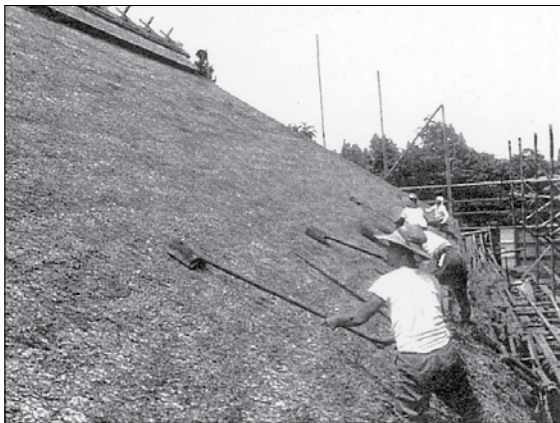
9 屋根面整形(かんぎ) Regulation of roof side
