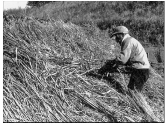
4 平葺き Thatching of field
