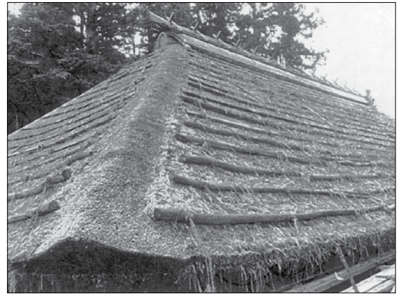
8 葺き上げ完了 Thatched completion
