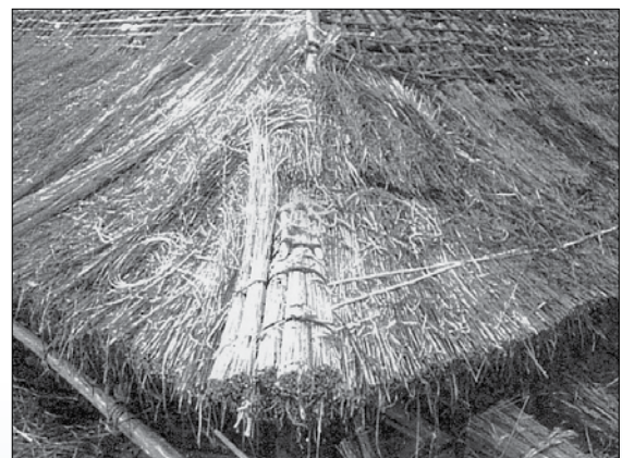
6 隅部軒付け(水切茅) Corner of eaves
