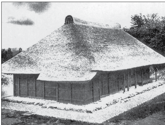
7 茅葺き工事完成 Thatching completion
