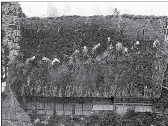
1 屋根剥き Removal of old straw
