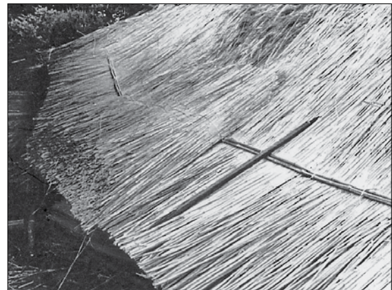
4 軒付け(水切りヨシ) Thatching of eaves
