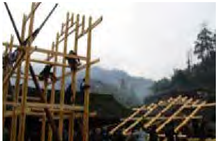
Pic 13: Pull the timber frame up
