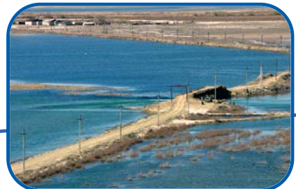
Rayy Lake and Zhalanash pumping plant, Kazakhstan © UNESCO/Zhanat Kulenov
