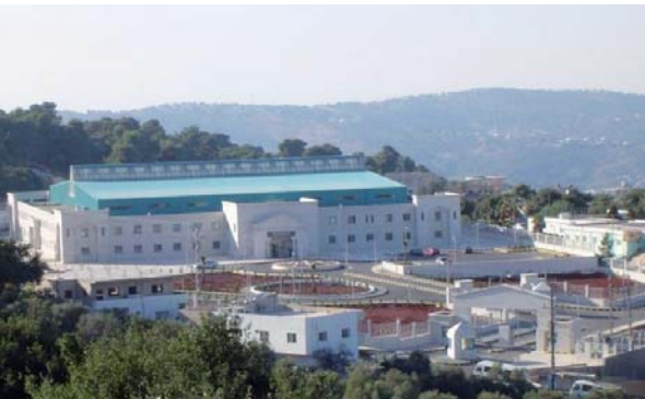
The SESAME building at Allan (Jordan), some 35 km northwest of Amman, where installation of the accelerator complex has begun. Financed by Jordan, the building has been designed by civil engineers from Al-Balqa' Applied University. It was officially inaugurated on 3 November 2008.
