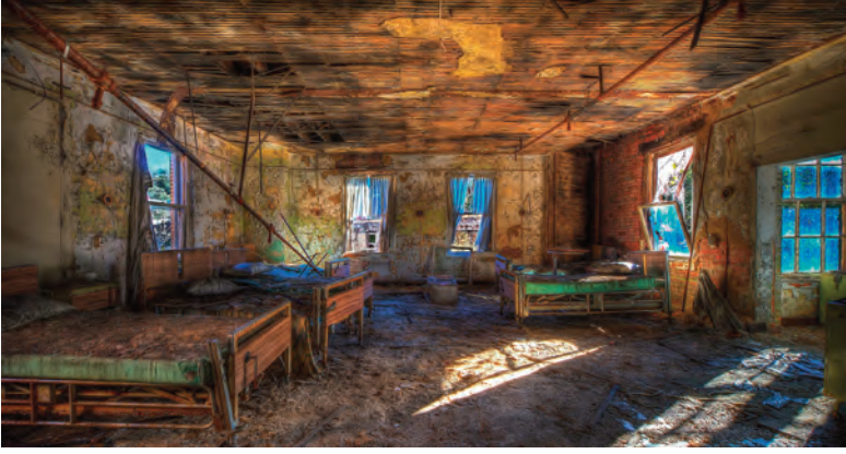
Abandoned hospital in Pittsburgh (USA) © Brook Ward/Flickr.com*
