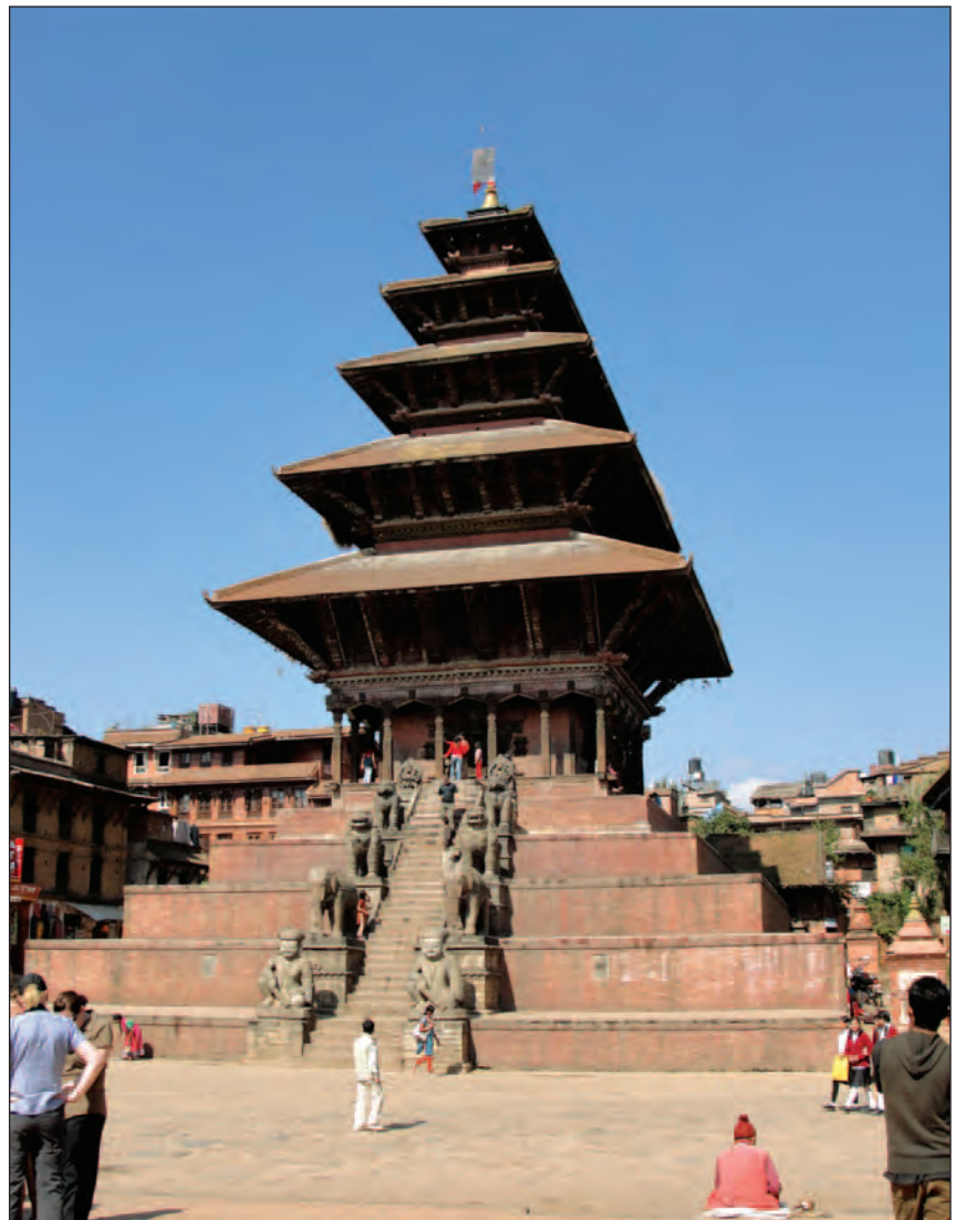
Figures 2: Nyatapola temple in Bhaktapur after renovation; top floor was damaged in 1934 earthquake.
