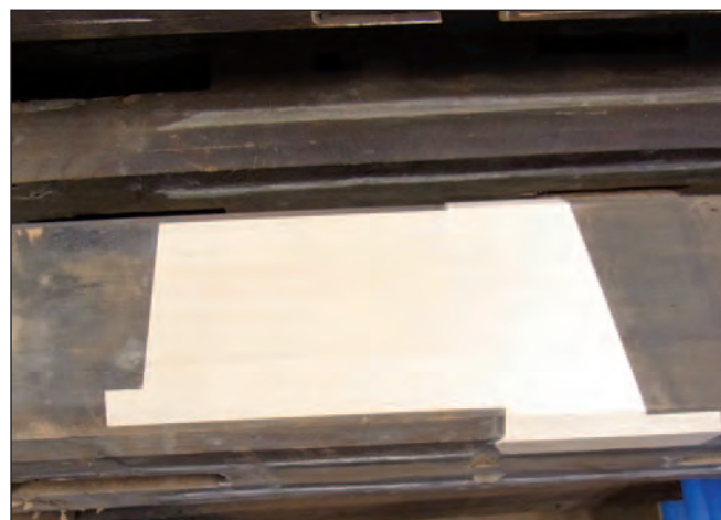
Figure 1: Repair of an old member through woodworking in Japan
