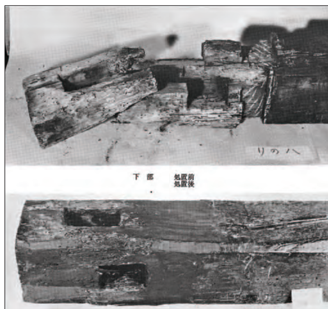
Figure 2: Repair of a pillar (Hakogi Farmhouse)
