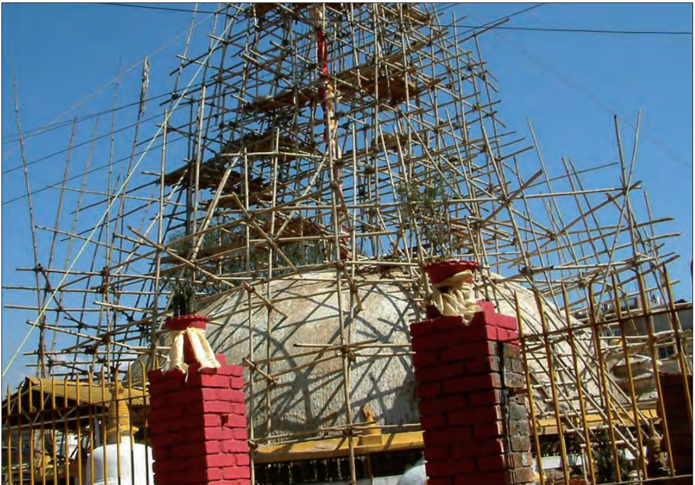
Figure 4: Chabel Chaitya restoration
