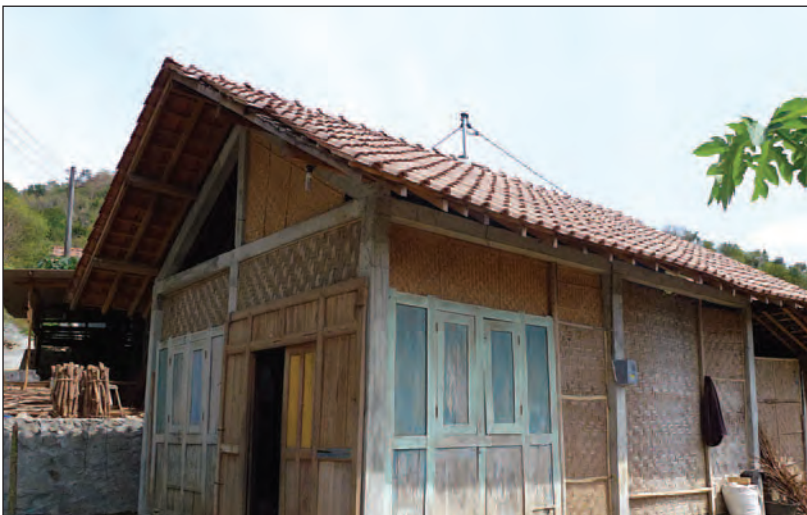
Figure 7: Parts of an old limasan in a new house in Jatirejo, Yogyakarta (2012)
