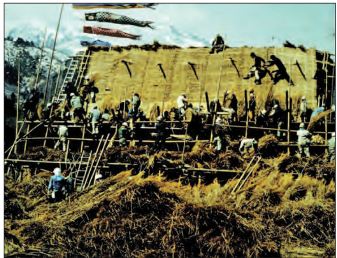
Figure 13: Roof thatching cooperative work at Shirakawa
