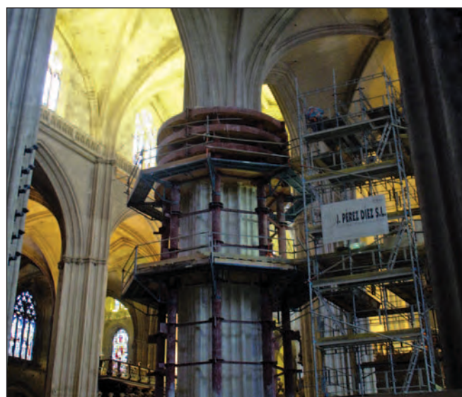
Figure 3: Replacement of pillars in Seville Cathedral
