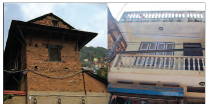
Figure 7: Transformation of sloped roof in traditional building to the flat roof of recent developments
