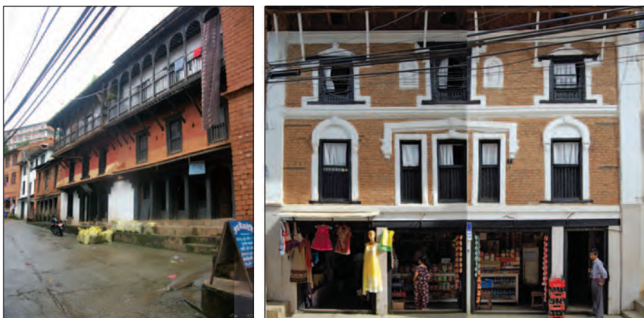
Figure 3 & 4: Traditional Newari Houses in the core of Tansen display the authentic architecture of Tansen
