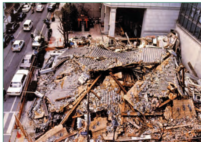
Figure 9: House No 15 after Kobe earthquake
