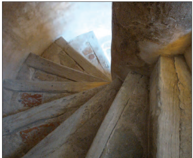
Figure 9: The current steps of the building are very narrow and high.
