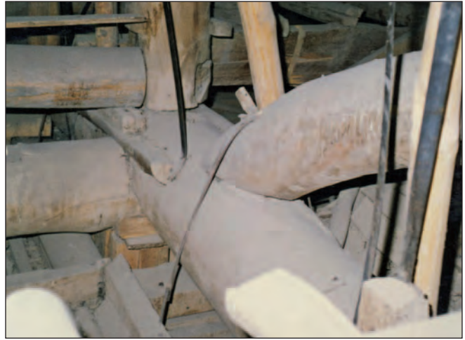
Figure 3: Wooden beams and trusses
