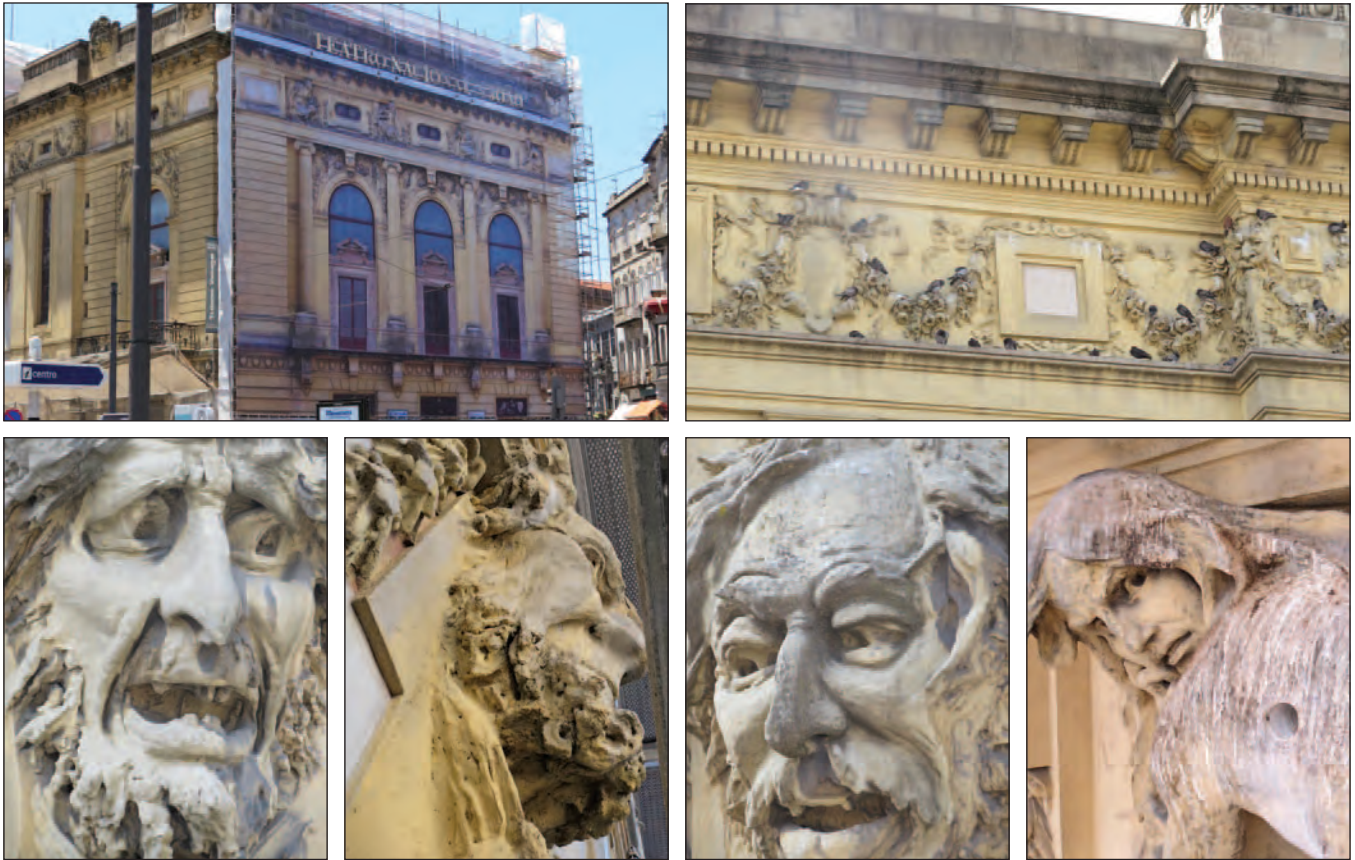
Figure 2 – Façades and reinforced concrete decorative elements of the São João National Theatre.
