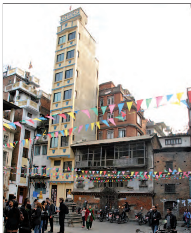
Vulnerable structures, Itum Bahal, Kathmandu
