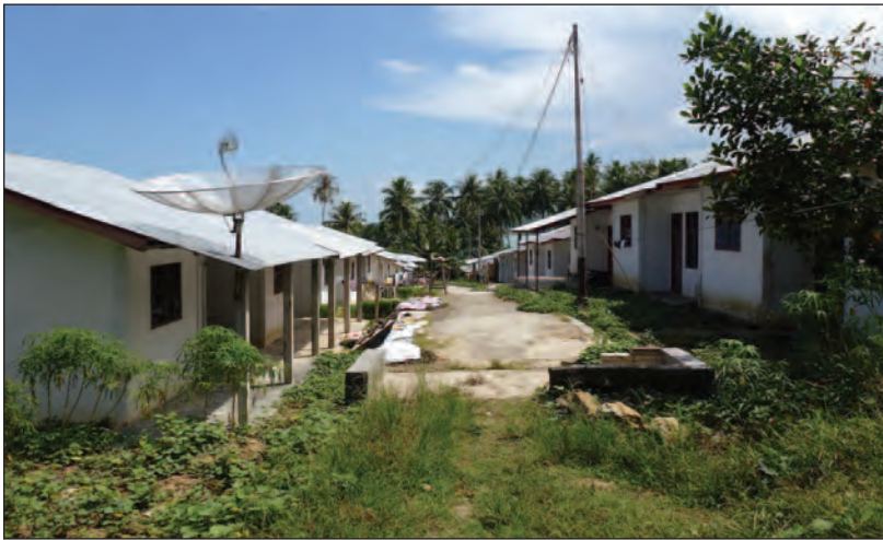
Figure 5: The BRR settlement at Sondregeasi, South Nias (2012)
