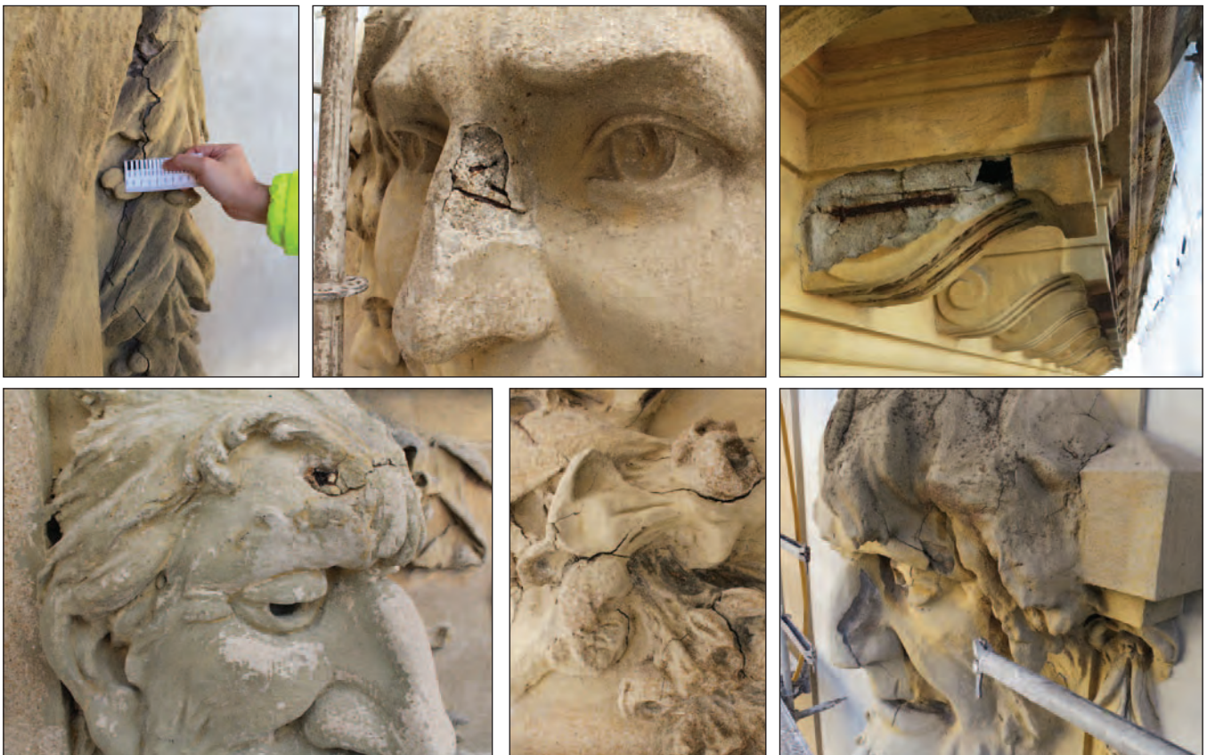
Figure 3 – Examples of damaged reinforced concrete decorative elements of the façades of the São João National Theatre.
