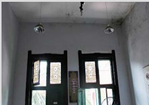
Figure 56: Window frames of Kedai Seni Jakarta remain in their original state
