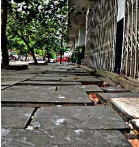
Sidewalk on Kalibesar Barat Street
