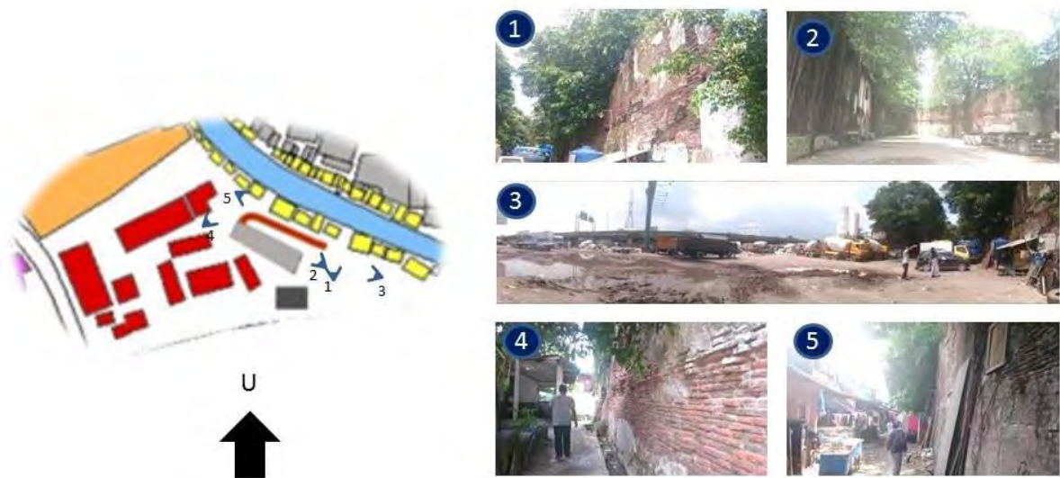
Figure V.6. The Old City Wall Source: Field Observation, 2015
