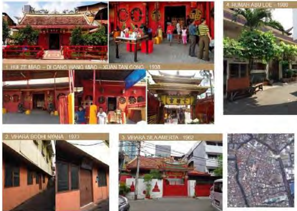
Figure II.29. Confucian Temple and Buddhist Vihara Sub-ethnic Communities of Hakka & Konghu Source: Field Observation, 2014
