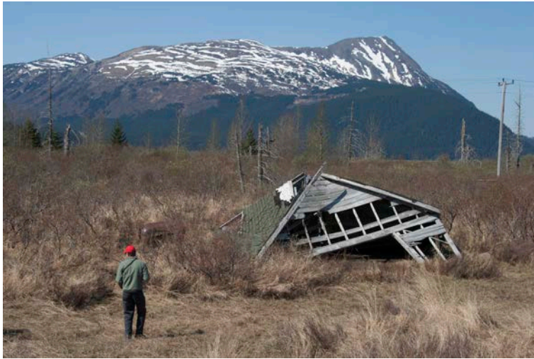
Coseismic subsidence produced in the Alaska 1964 Earthquake (Portage Garage, Alaska)
