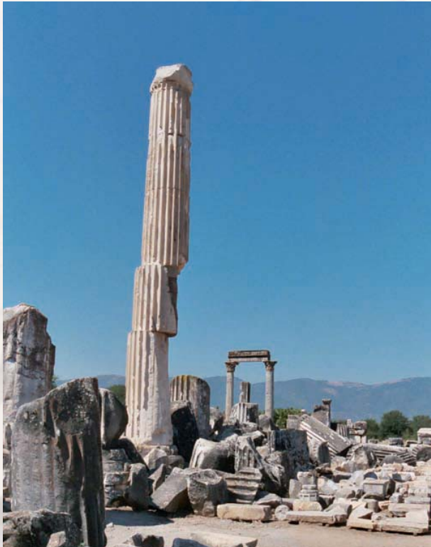
Typical earthquake-related structural damage pattern: displaced drums of a column keystone in the Temple of Aphrodite in the Roman city of Aphrodisias in southwest Turkey, near the modern town of Geyre, west of Denizli. © Manuel Sintubin
