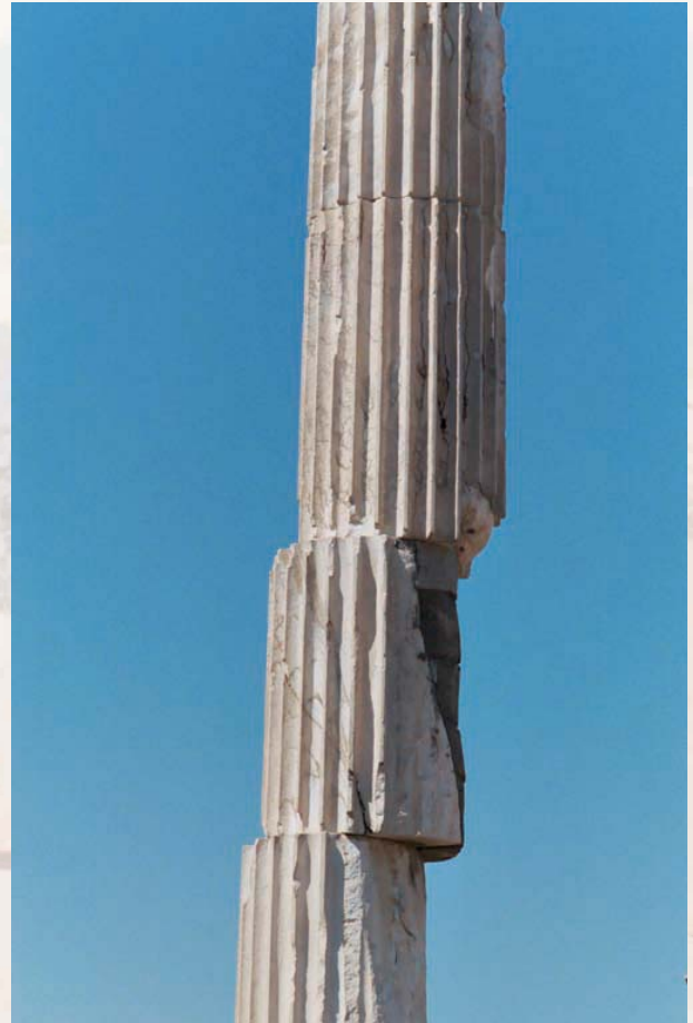
Typical earthquake-related structural damage pattern: displaced drums of a column keystone in the Temple of Aphrodite in the Roman city of Aphrodisias in southwest Turkey, near the modern town of Geyre, west of Denizli. © Manuel Sintubin
