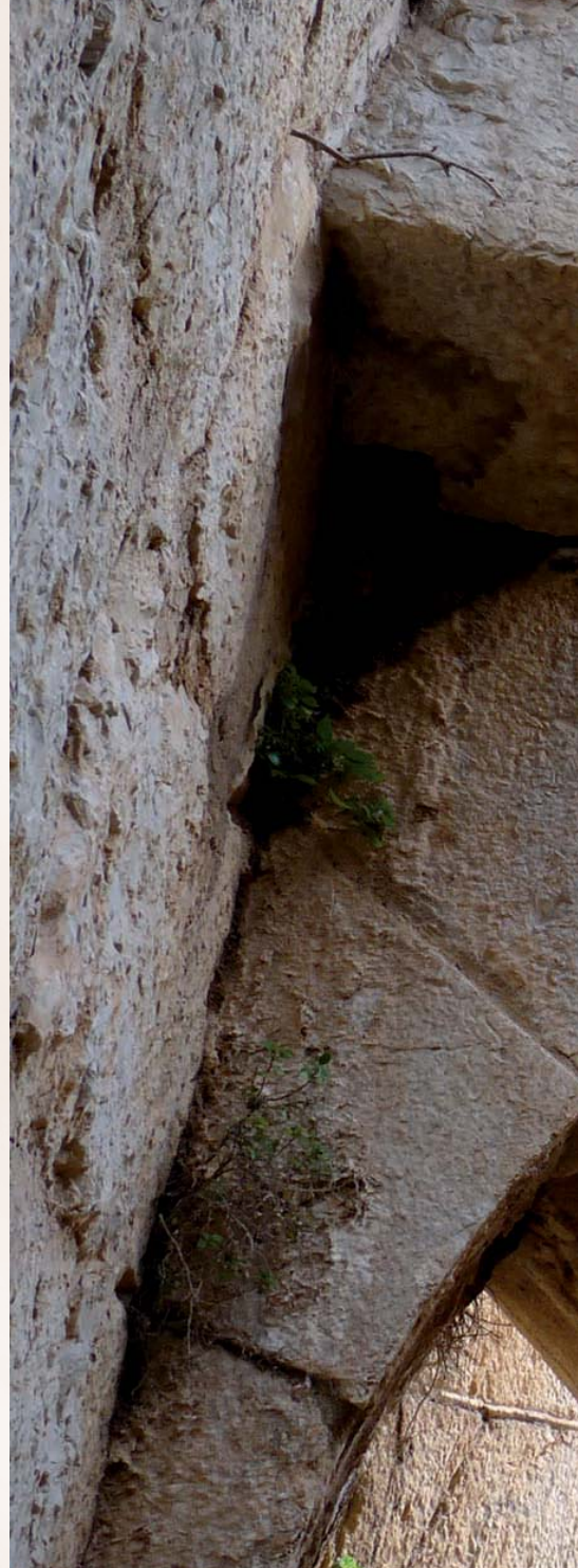
Typical earthquake-related structural damage pattern: dropped keystones in an arch in the medieval Nimrod Fortress, or Kal'at Al-Subayba on the Golan Heights. © Manuel Sintubin
