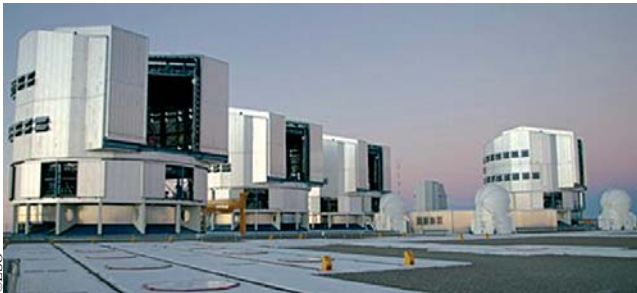
The Paranal Observatory in northern Chile consists primarily of the Very Large Telescope of the European Southern Observatory. There are four telescopes in all, each measuring 8 m in diameter, or the equivalent of a large 16-metre telescope. The VLT is arguably the most sensitive instrument in the world. For the past three to four years, it has been making observations of unprecedented quality
