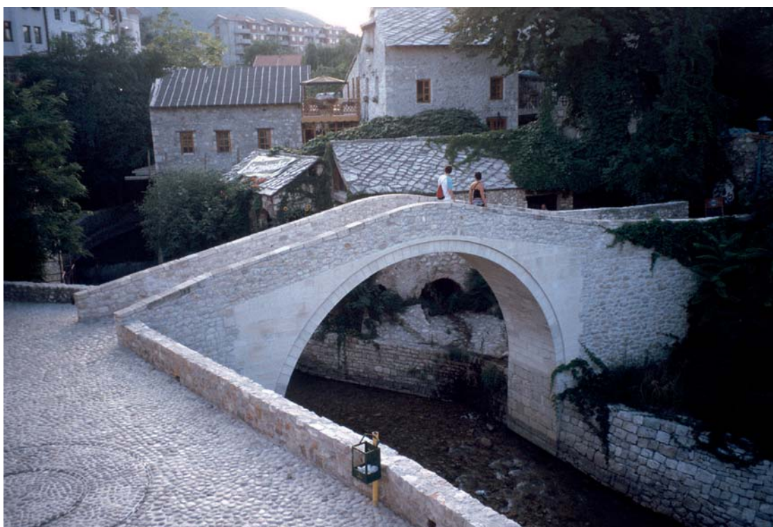
4.16 Mostar Bridge, Bosnia and Herzegovina (© UNESCO)
