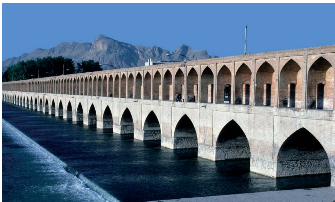
3.20 Siyehpol Bridge, Isfahan (© G. Degeorge)
