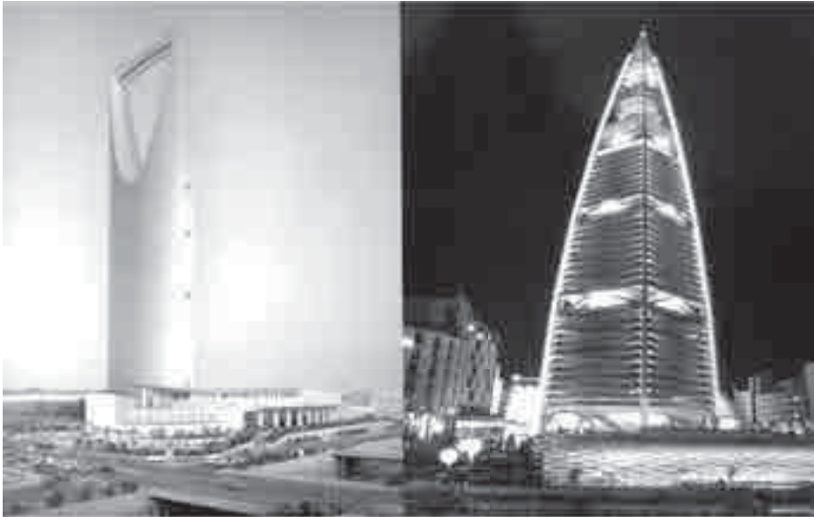
VI-1.1 Kingdom Tower (left) and Faysaliyyah Commercial Tower and Hotel (right) in Riyadh, Saudi Arabia
