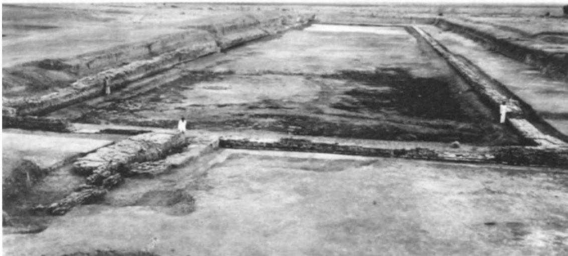
FIG. 10 Lothal: Brick structure, known as a dockyard, with a spillway in the foreground.
