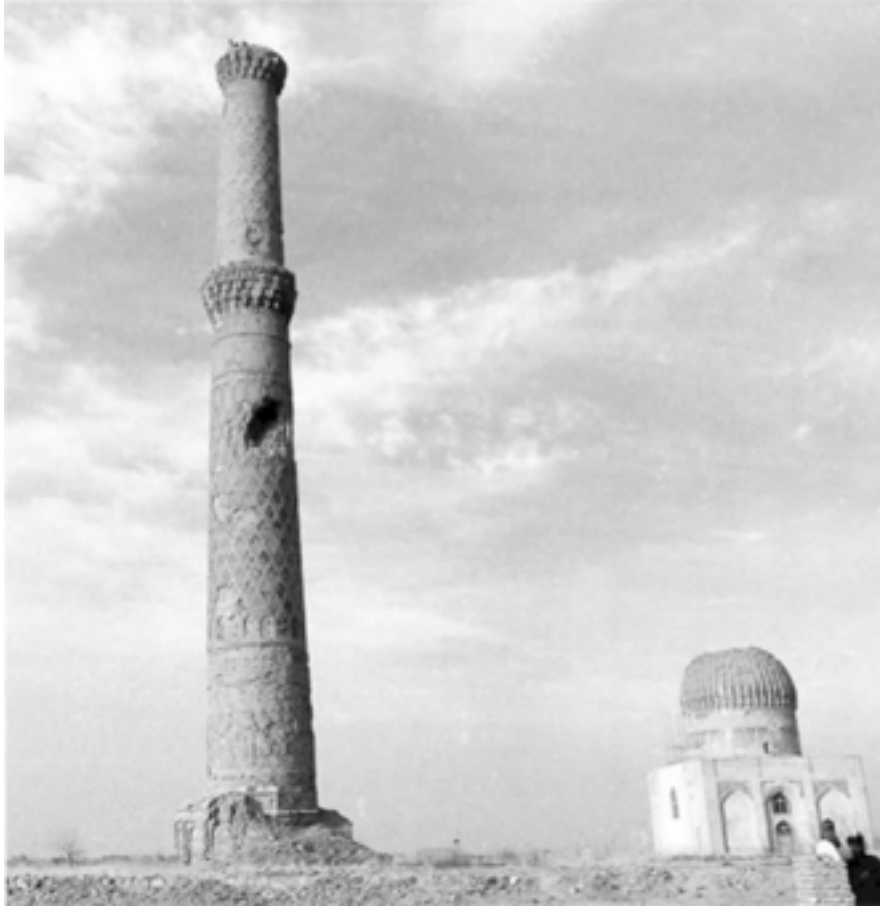
Fig. 10. Herat. Minaret of the madrasa of Gawhar Shād (mid-fifteenth century). (Photo: Courtesy of C. Adle.)
