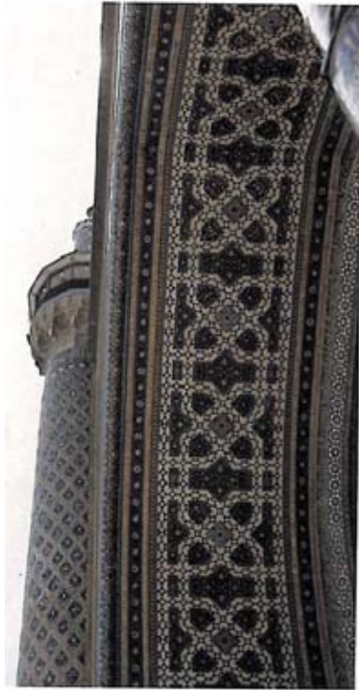
Fig. 39. Mashhad. View of a minaret from an aiwān . (Photo: Courtesy of H. R. Zohoorian.)
