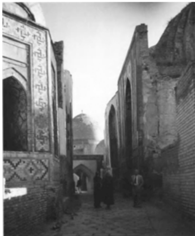
Fig. 50. Samarkand. Shah-i Zinda complex. View of the mausoleums alongside the path. (Photo: Courtesy of I. Iskender-Mochiri.)
