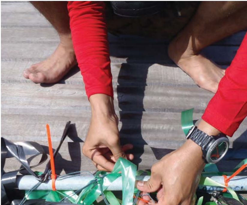
Like debris nets and geotextile, it is easier to install the artificial seagrass on the seabed when it is fixed to a heavy iron pole. © UAD, Thailand
