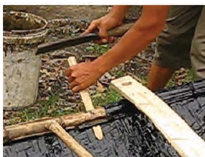
Example of a construction sequence documented step by step. Mr. Toan Huyen's boatyard, Huong Hoc village, Quang Ninh province. © Charlotte Minh-Hà Pham
