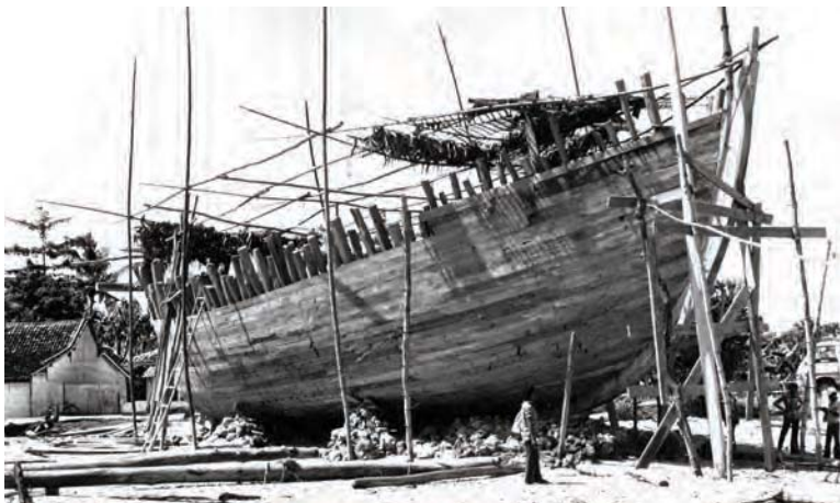
This lete-lete under construction in Gayam, Sapudi is a good example of a perahus. This contemporary design has been influenced by Dutch boat building in the Madura region. © Kurt Stenross
