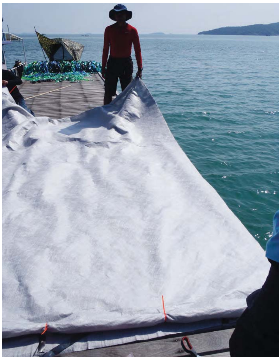
Geotextile is being fixed to a heavy iron pole before taken into the water, which reduces the buoyancy. © UAD, Thailand
