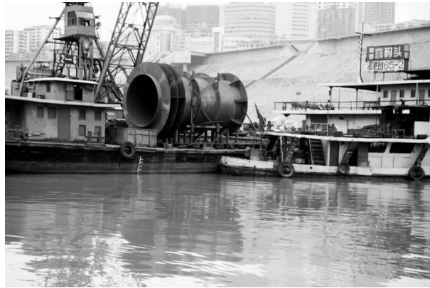
Fig. 28 Transport of embedded pipe joints
