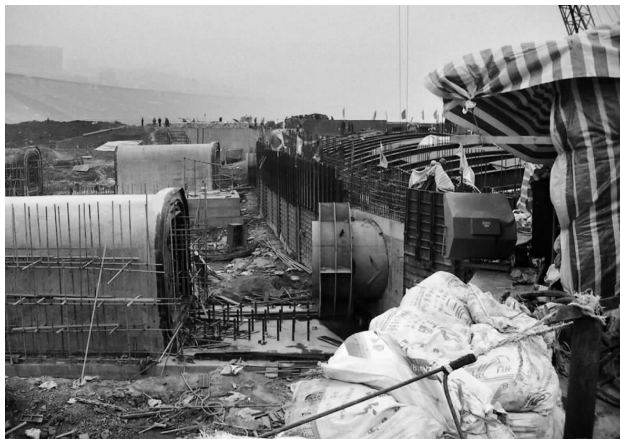
Fig. 36 Construction of the horizontal traffic gallery at up and downstream ( IV )
