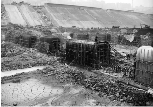
Fig. 35 Construction of the horizontal traffic gallery at up and downstream ( III )
