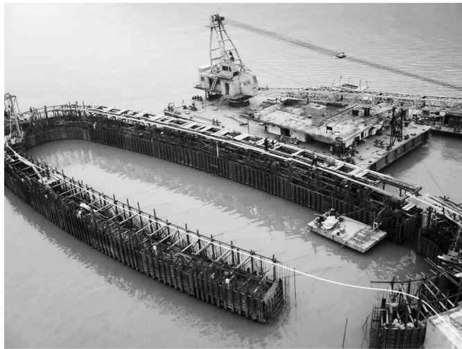
Fig. 27 Construction of 3.5m thick guide wall in the protection structure
