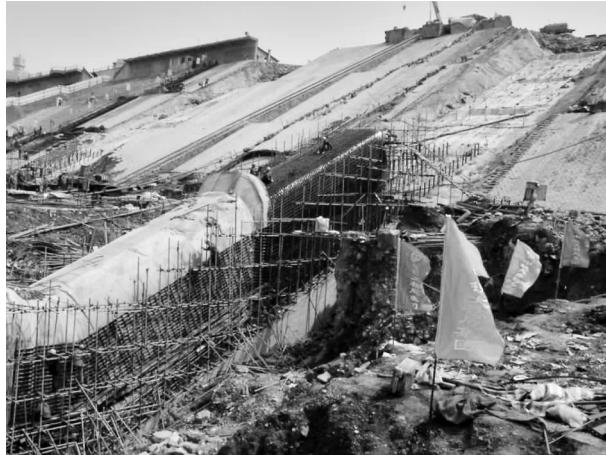
Fig. 40 Construction of the slope traffic gallery (IV)
