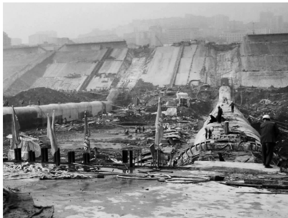
Fig. 39 Construction of the slope traffic gallery (III)
