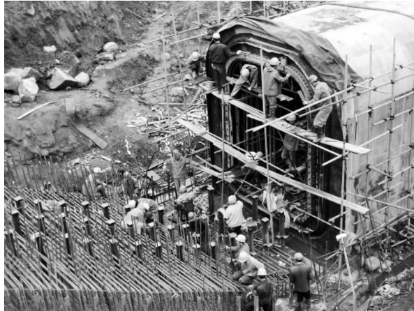
Fig. 38 Construction of the slope traffic gallery (II)
