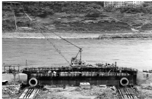
Fig. 29 Completion state of the guide wall
