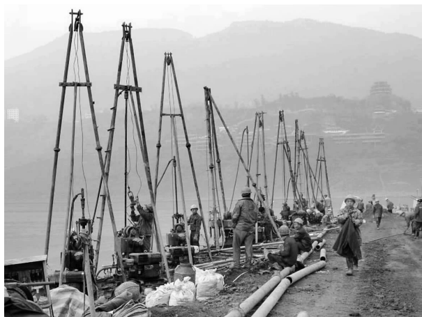
Fig. 30 Cofferdam construction
