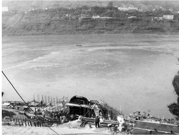
Fig. 37 Construction of the slope traffic gallery (I)
