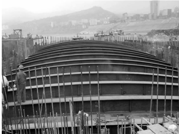
Fig. 48 Steel frame in dome
