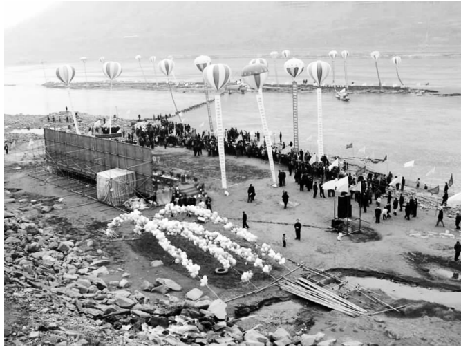
Fig. 22 Start of the in-situ underwater protection project for Baiheliang
