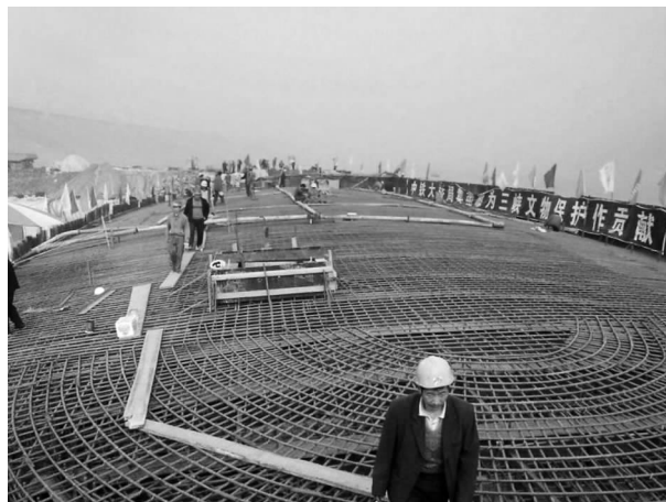
Fig. 49 Steel meshes of reinforced concrete in dome
