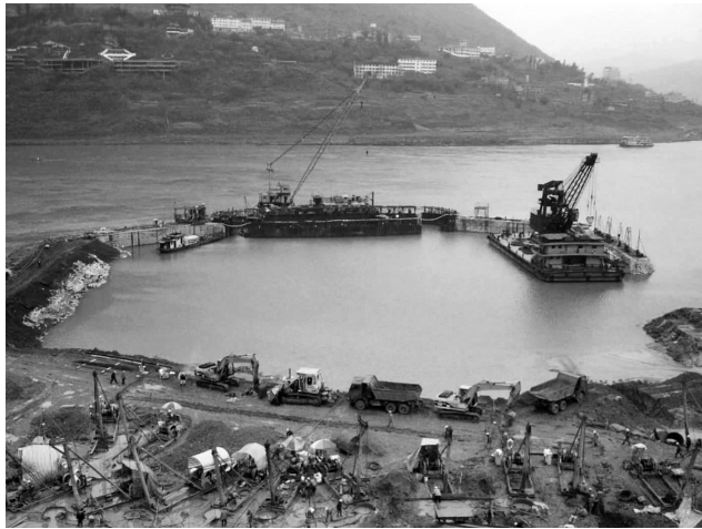
Fig. 31 Approaching completion of the cofferdam
