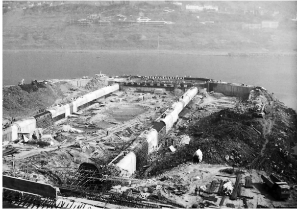
Fig. 34 Construction of the horizontal traffic gallery at up and downstream ( II )
