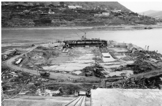
Fig. 32 Construction field after closing cofferdam
