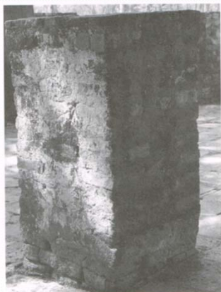
23) Brick pillar in Wat Sri Chum just after application of the new type biocide
