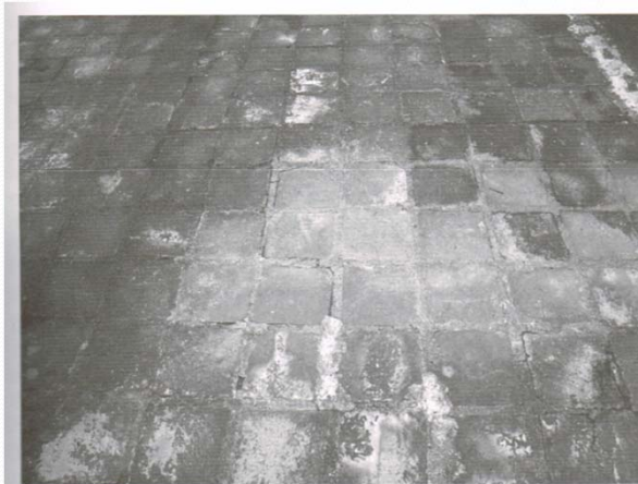
27) Part of brick floor at Wat Sa Si six months after application of the new type biocide
