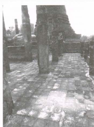
26) Part of brick floor at Wat Sa Si six months after application of the new type biocide
