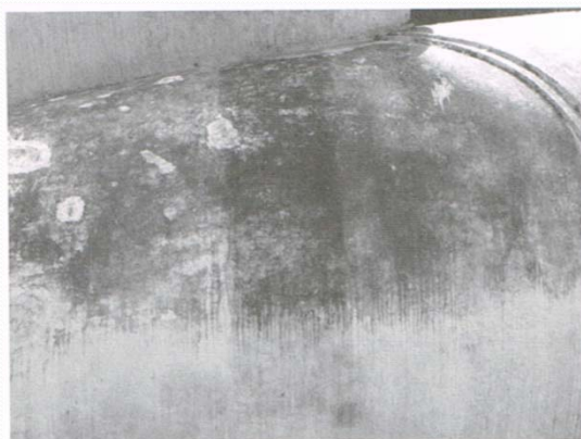
19) Part of giant Buddha statue just after application of the new type biocide
