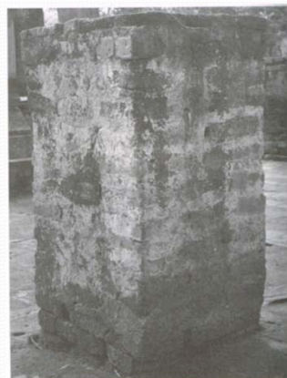
24) Brick pillar in Wat Sri Chum six months after application of the new type biocide
