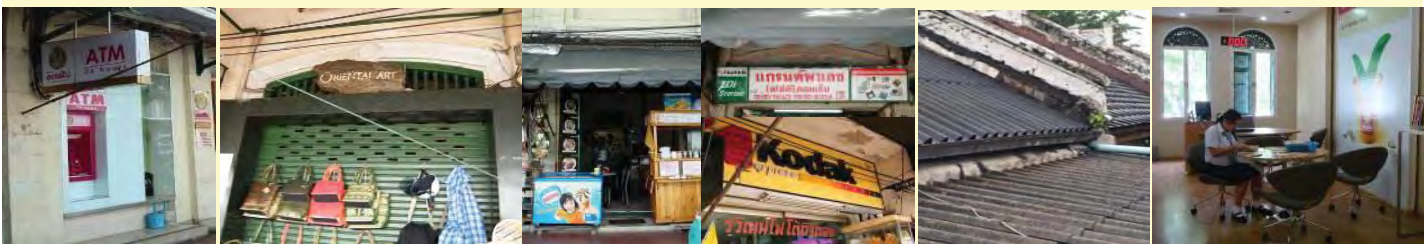
Illegal building alterations
