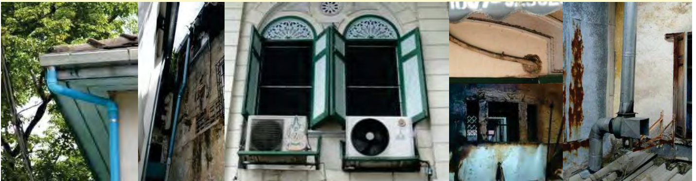
Inappropriate installment of facilities and wires
