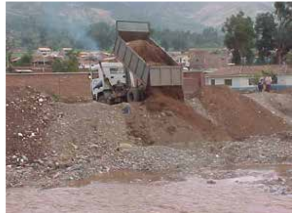
Figure 16. Discharge of cuttings into the Huatanay (San Juan de Dios, San Jerónimo, Cusco)
