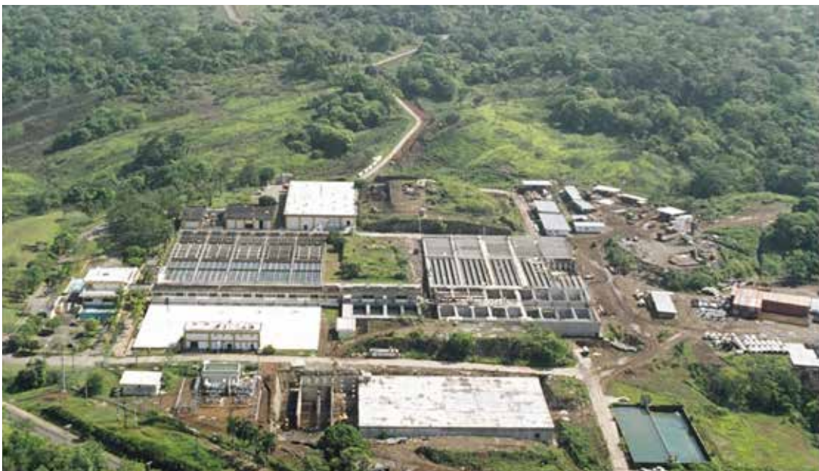
Figure 4. Chilibre water treatment plant with a capacity of 250 MGD, the largest in Panamá
