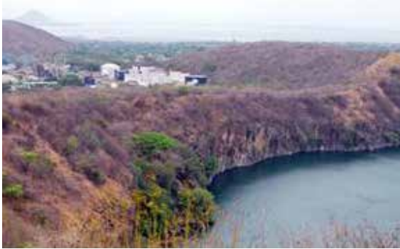
Figure 2.4 The Refinery on the North Bank of the Asososca Lagoon
