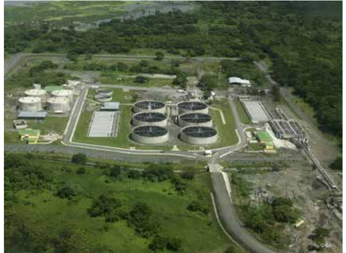
Figure 4.1 Modern Wastewater Treatment Plant for the City of Managua
