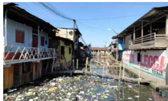
Figure 17. Iquitos, sewers in the neighborhood of Belén
