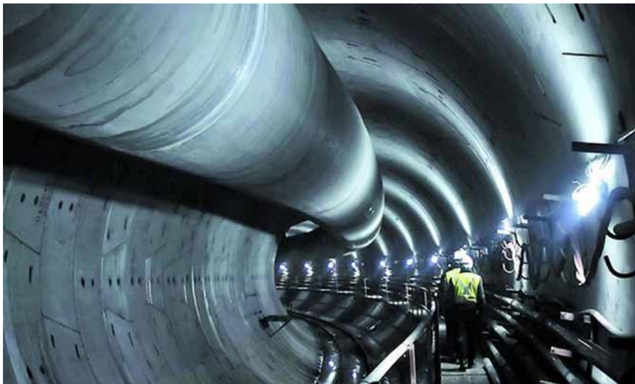
Figure 18. Construction of relief tunnels in the city of Buenos Aires
