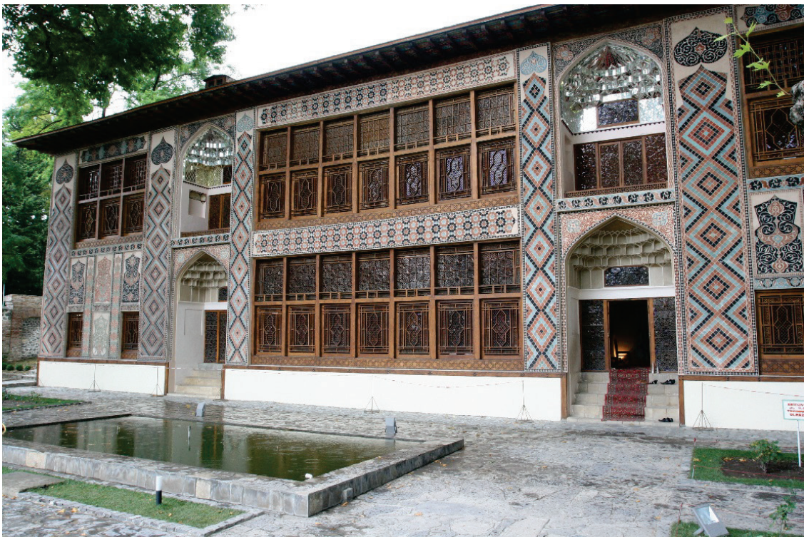
South façade of the Khan's palace
