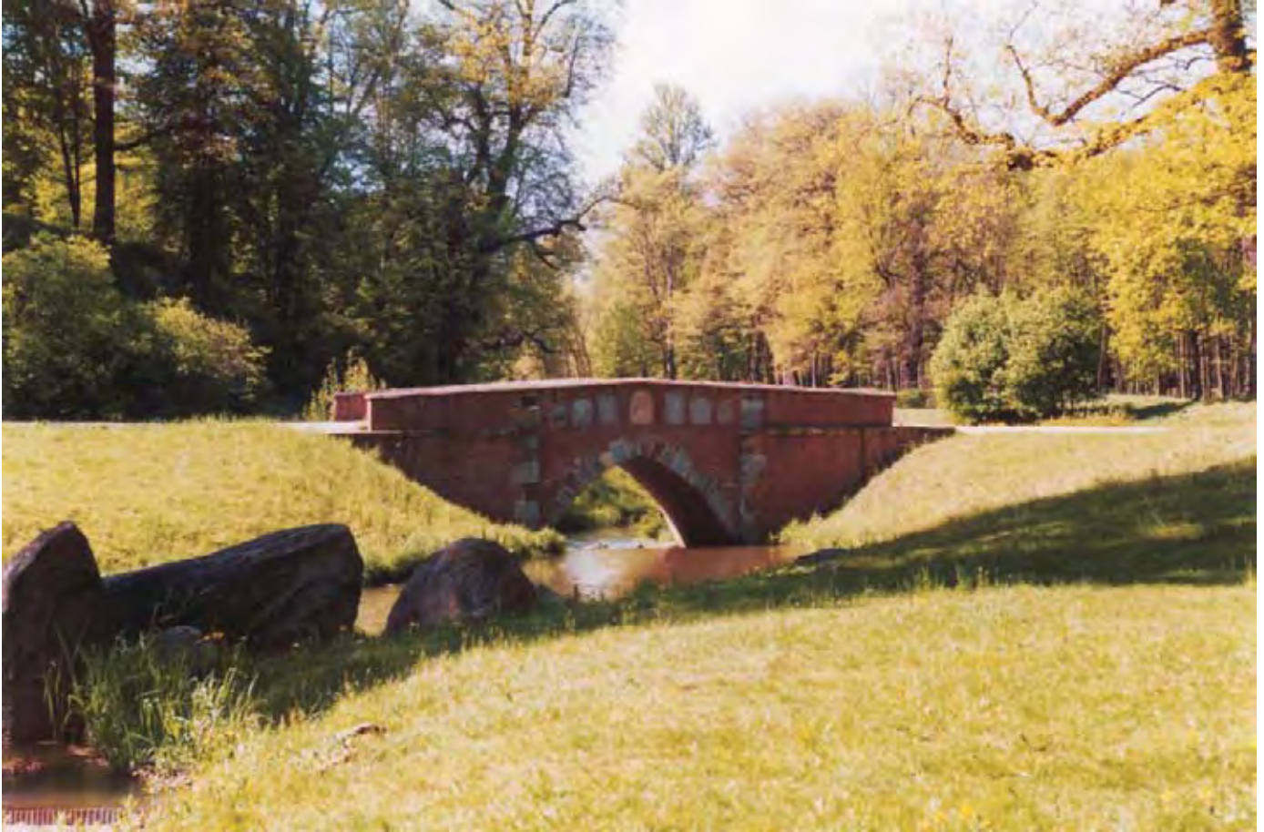
13. Bridge near the Oaks' Lake (German side)
