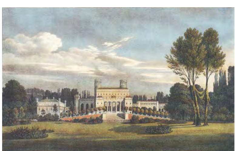
2. The Castle and the ramp seen from the Bowling Green
