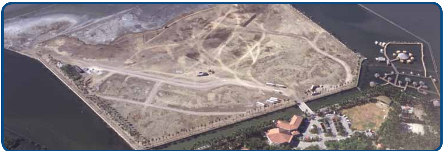
Land reclamation for tourist infrastructure development, the Philippines. Mark Spalding
